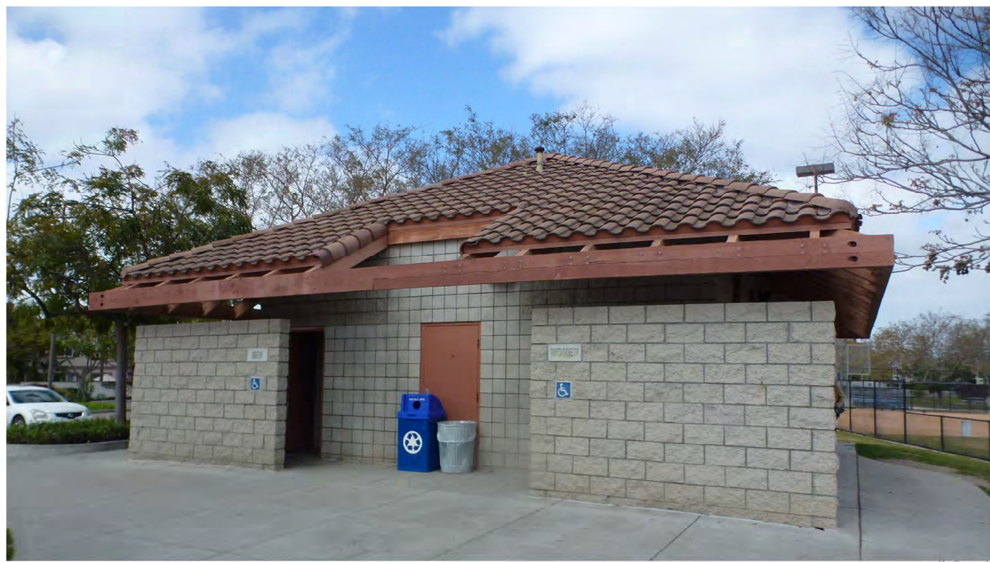
EXISTING RESTROOM BUILDING
