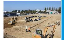
As part of Phase 1 of the Pure Water Program, the NCWRP is being expanded from a capacity of 30 mgd to 52 mgd. Early site work has focused on clearing areas where new facility components will be constructed. For example, cranes were used to relocate the first two steps of the Pure Water Demonstration Facility (ozonation and biological activated carbon filters) to make room for the new pump station. Construction is expected to begin in mid 2021.
