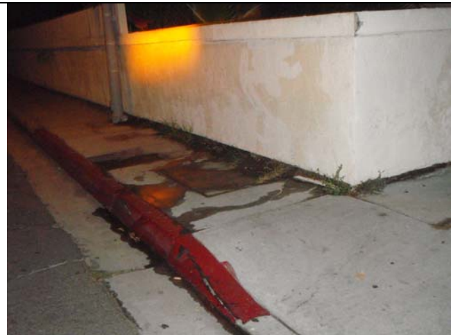
Figure 10. Sprinkler Runoff at Elizabeth Street and Logan Avenue
