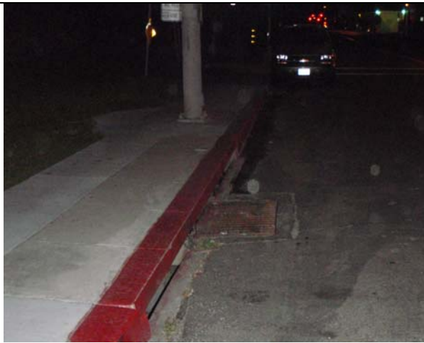
Figure 9. Storm Drain Inlet along East Side of 43 rd Street, South of Logan Avenue
