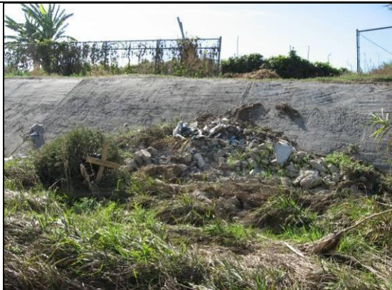
Trash and debris dumped through a break in a fence (observed January 2010).
