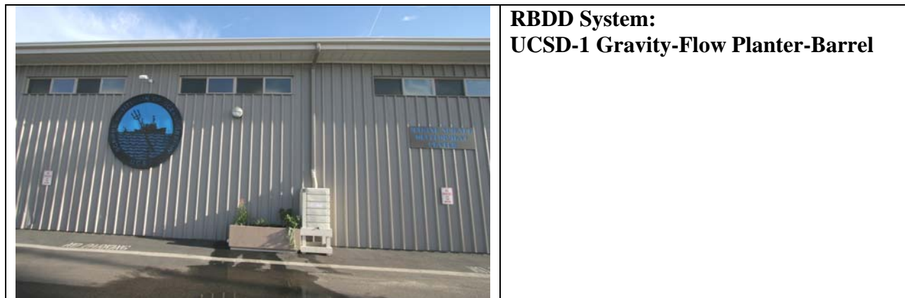
Figure 2-5. Scripps Institution of Oceanography Metalshop Building Downspout Disconnect Installation Photograph(s)
