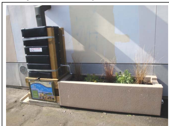
Figure 5-1. Complete Planter-Barrel System Ready for Operation
