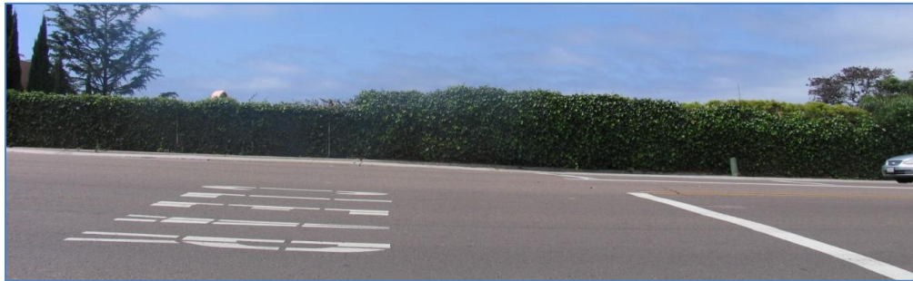
Picture 3399 - Charlotte Street Fence Overgrown with Ivy
