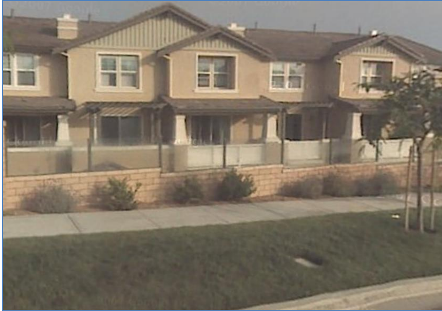
Example of cement block wall parapet with Plexiglas top. Parapet is on top of a retaining wall in 4S Ranch area
