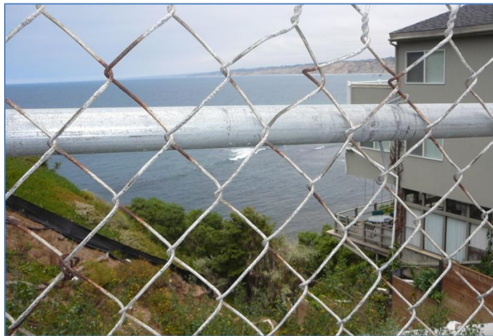
Picture 3957- View through Opening in Fence
