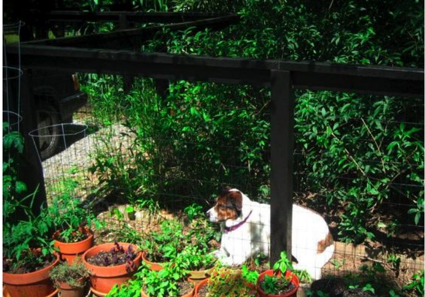
Example of a 42-Inch High Wood Fence with Wire Fabric
