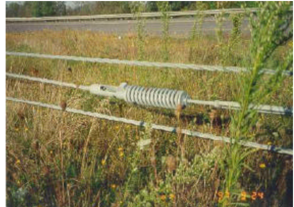
Three-Cable barrier installed in Oregon.
