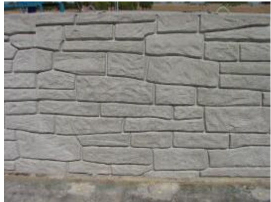
Type 60 Concrete Barrier with aesthetic treatment
