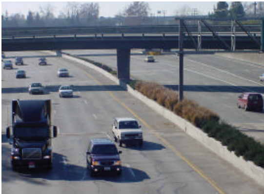
This is a concrete barrier with paving to the face of the barrier and landscaping in the median.
