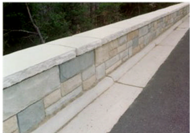
This guardwall is installed on the Federal highway system in the East Coast.
