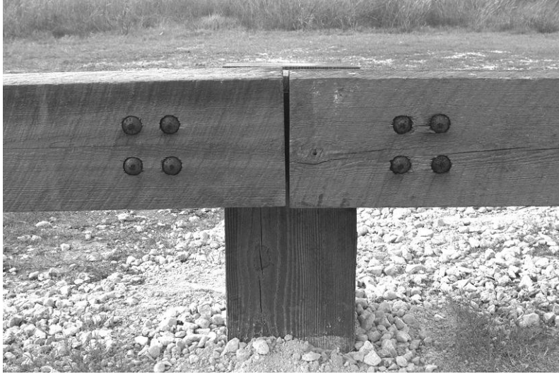
Timber Guardrail Post Detail
