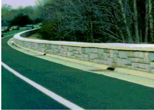
A Precast Concrete Guardwall Installation
