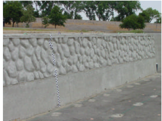
Shown here is rock cobble pattern with 610 mm of light sandblast on the bottom of the barrier.
