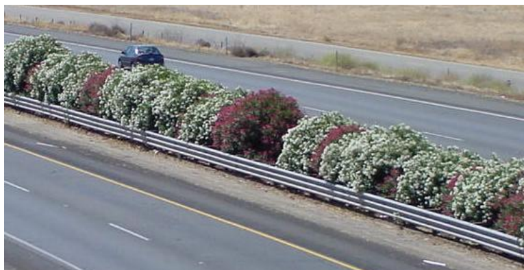
Thrie Beam Barrier along a highway
