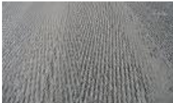
Diamond Grooved Pavement
