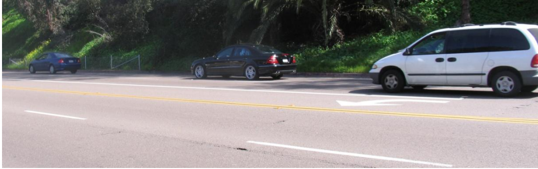
Picture 2356 - Left-Turn Pocket in the Median
