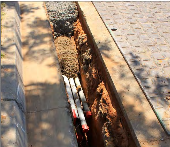
Recently installed utilities.
