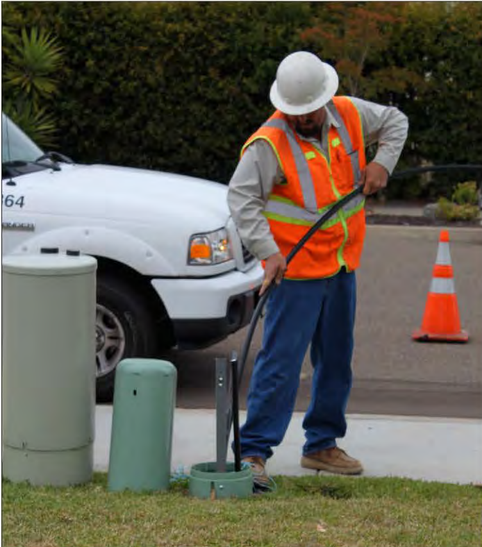
Crew member installs the last of the underground cabling for the area.
