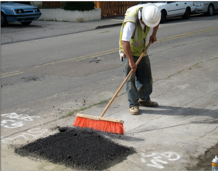
Construction crew member finalizes trenching repair with an asphalt seal.
