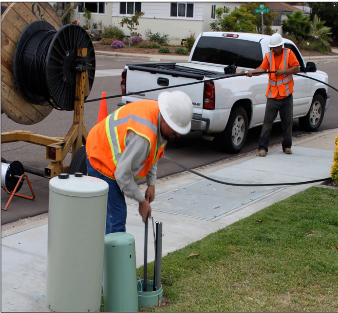
Construction crew members install utility cabling.
