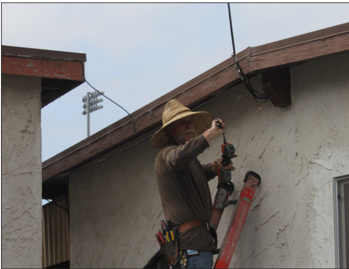
An AT&T crew member begins to remove the overhead utility lines.
