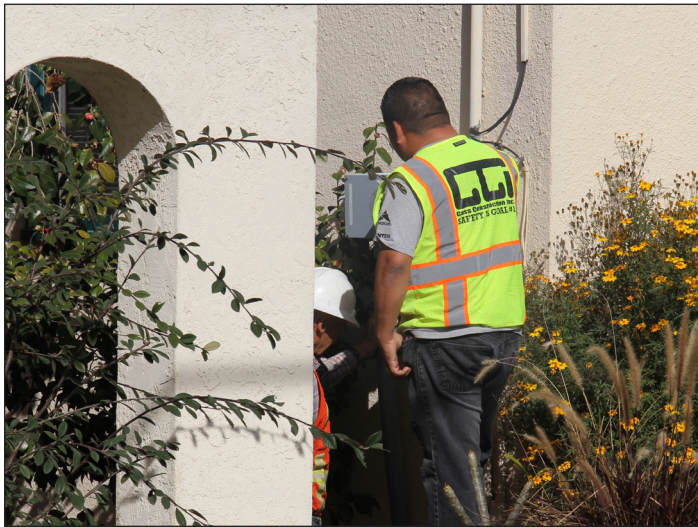
Crews evaluate recently installed underground conduit lines.
