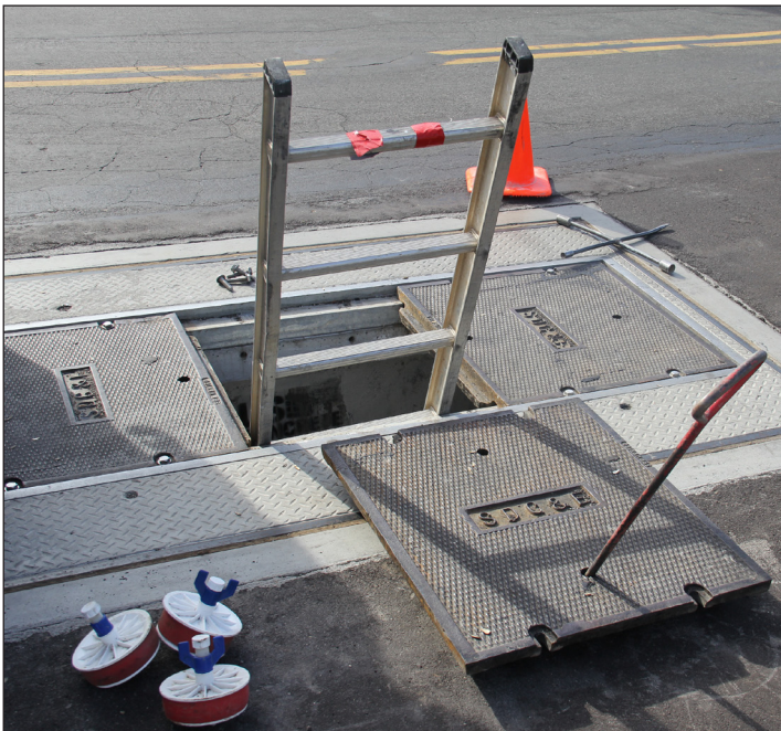
A subsurface SDG&E utility vault.
