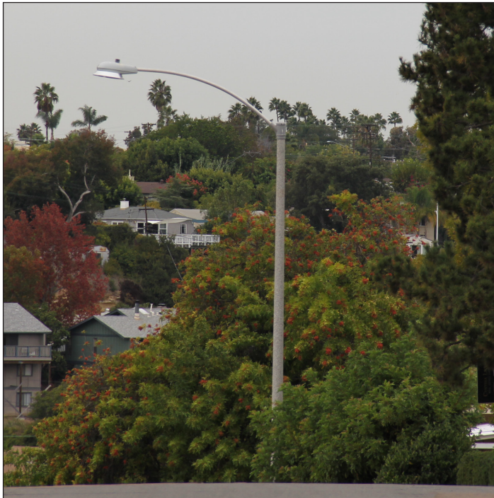
Crews will start installing streetlights, like the one pictured above, this month.
