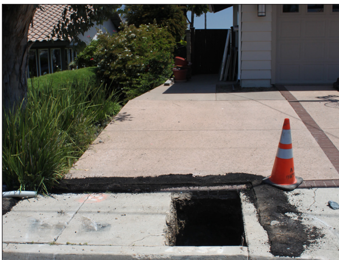
Customer service trenches house conduit lines from the street to the resident’s electrical panel.
