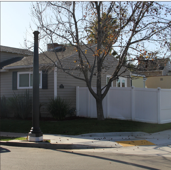
Acorn streetlights continue to be installed throughout the project block.
