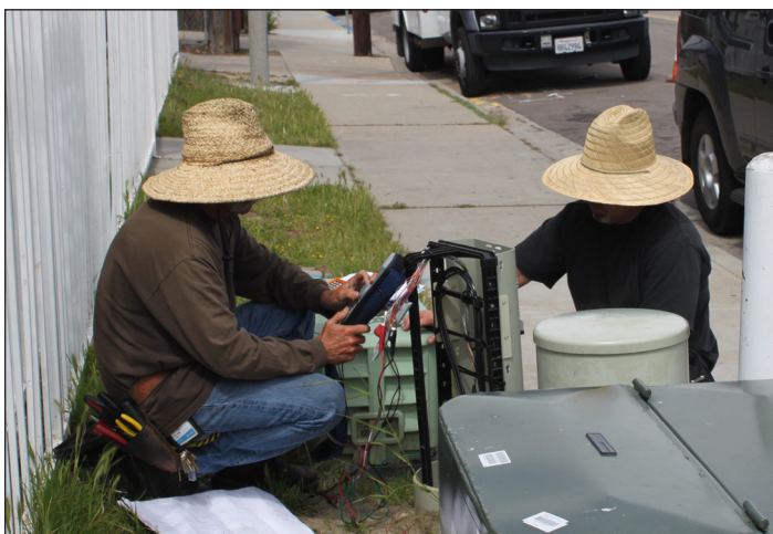
AT&T crew members work on a recently installed pedestal box to check that their cut-over activities were successful.
