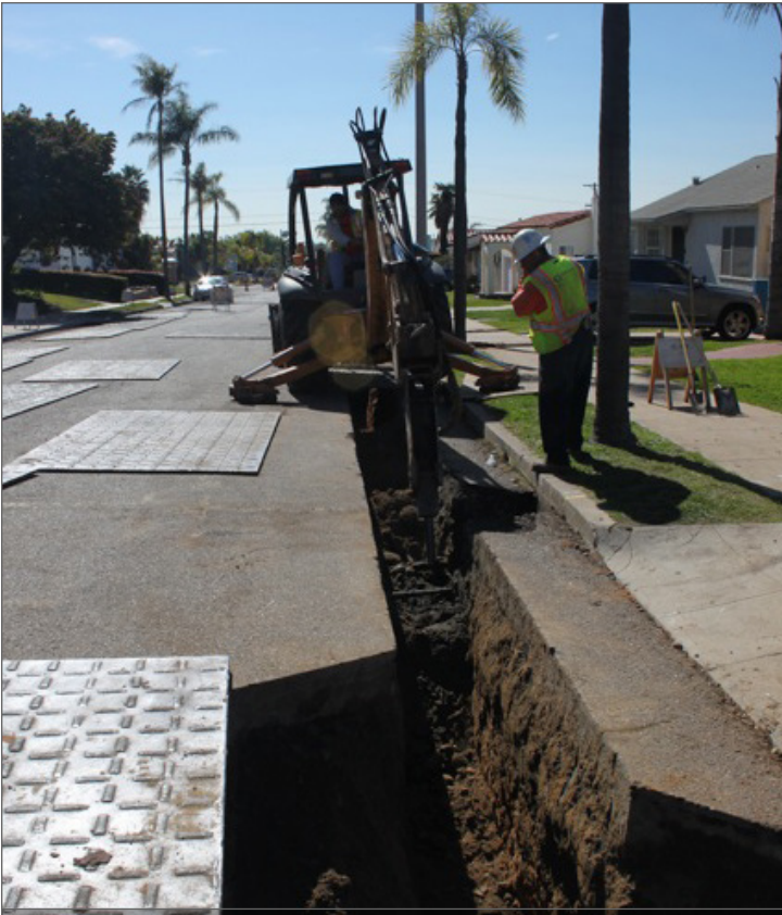
Crew members dig a mainline trench for the underground cabling.
