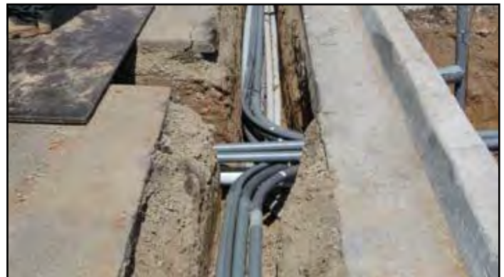
Example of Trenching with new underground conduit
