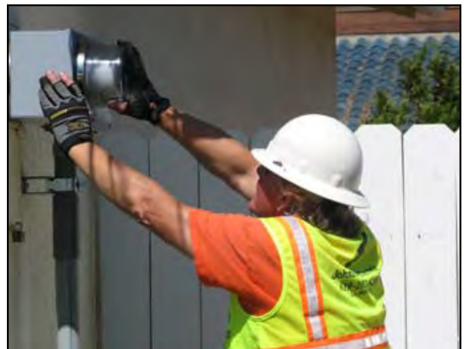
SDG&E crew member prepares an electric meter panel to accept the new underground service
