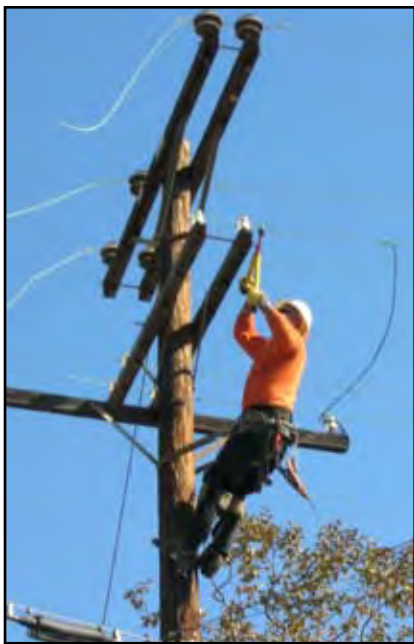
SDG&E crew member removes overhead lines
