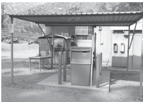
Despite almost everything around it being singed or burned, miraculously the gas pump station at El Capitan Reservoir survived the fires.
