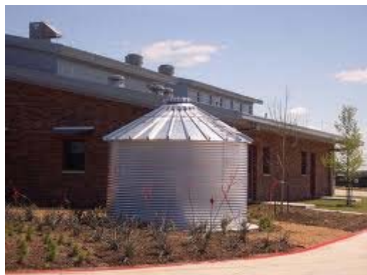
Figure 2. Large cistern on a commercial property
