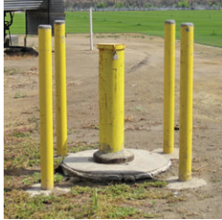
Groundwater Monitoring Well
