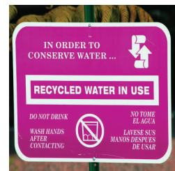
Typical signage indicating non-potable recycled water in use
