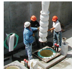
Groundwater Well Installation
