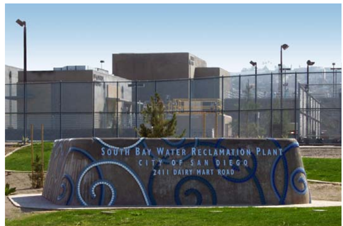
South Bay Water Reclamation Plant
