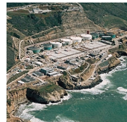
Point Loma WWTP
