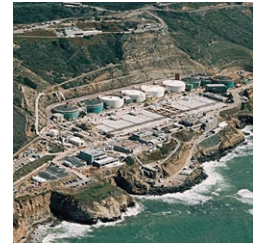
Point Loma WWTP
