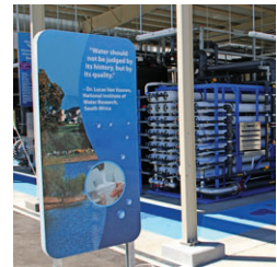
City of San Diego's Water Purification Demonstration Project
