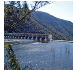
Lake Hodges Dam
