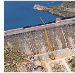
San Vicente Dam Construction
