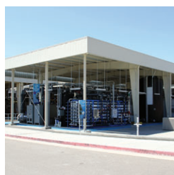
City of San Diego's Water Purification Demonstration Project
