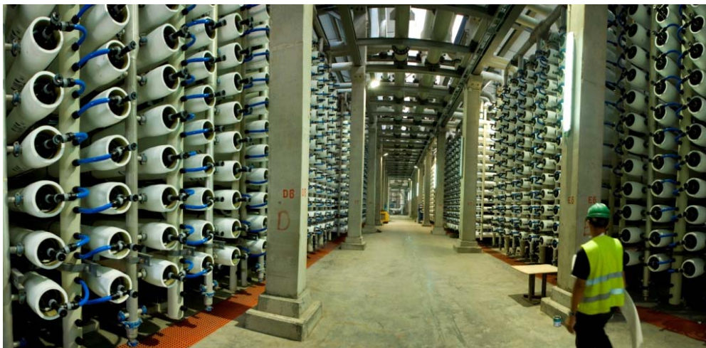
Figure 1. Treatment membranes for ocean desalination.
