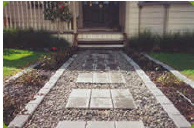
Example of Porous Paving
