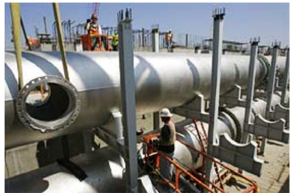
CHARLIE NEUMAN / Union-Tribune The Orange County Water District's plant under construction in Fountain Valley will produce five times more purified wastewater than the old factory.
