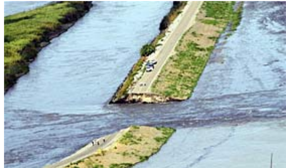
CRAIG SANDERS / The Stockton Record Water poured through this 300-foot break in the Bacon Island Road levee during the Jones Tract flood in June 2004. Flood repairs cost nearly $100 million.
