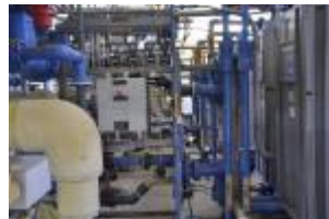
EDR (Electro Dialysis Reversal) area of the plant, where portions of the reclaimed water receive additional treatment for removal of dissolved solids.
