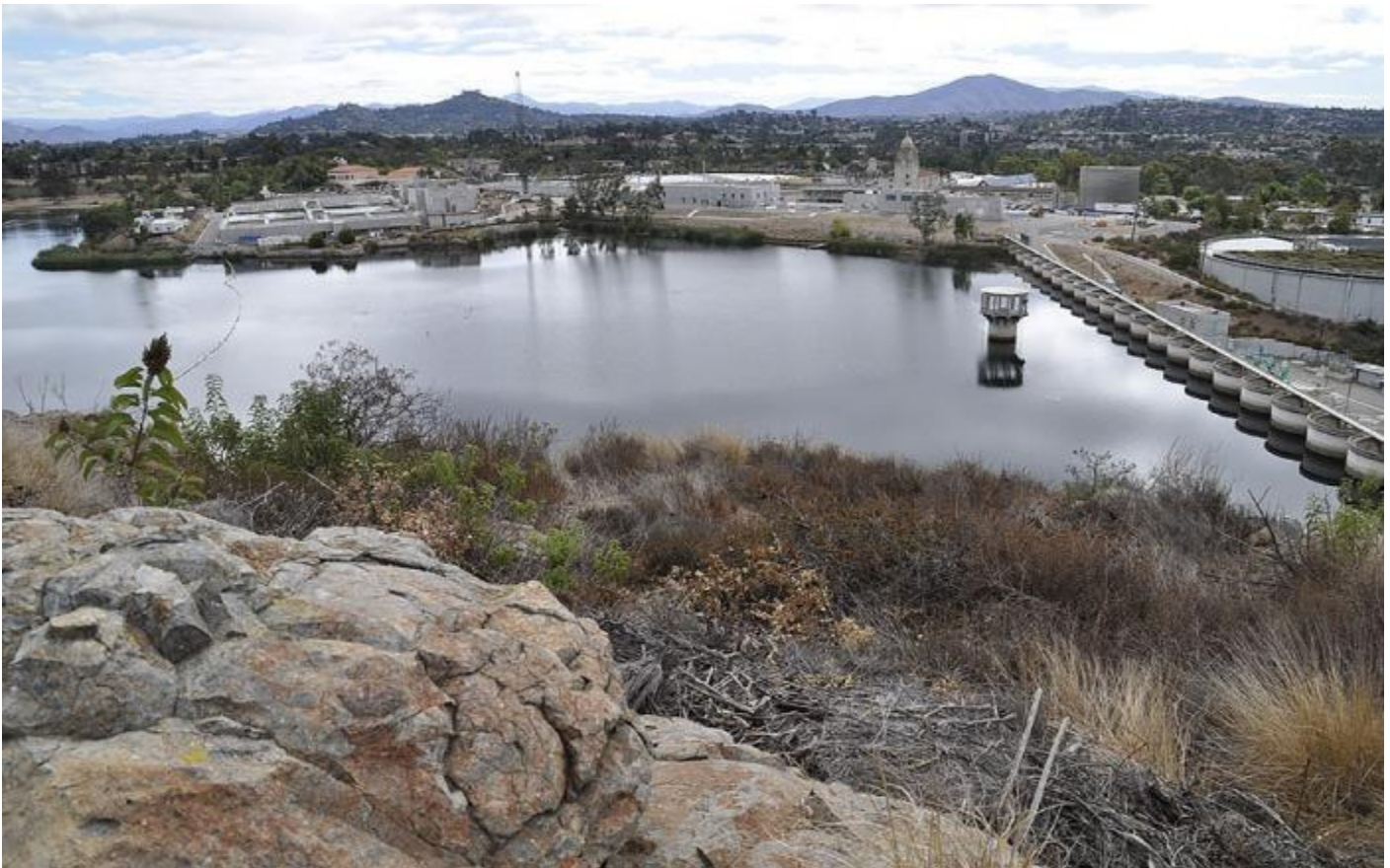
Alvarado Water Treatment Plant next to the dam at Lake Murray
