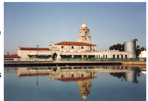
Alvarado Water Treatment Plant
