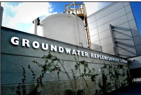
Orange County's water purification facility
