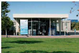
Advanced Water Purification Facility
