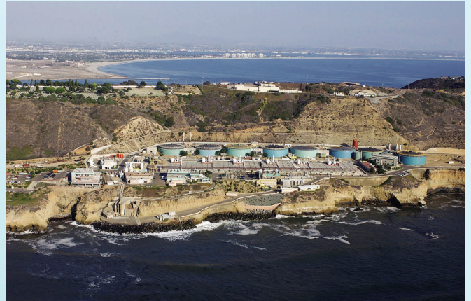
Point Loma Wastewater Treatment Plant
