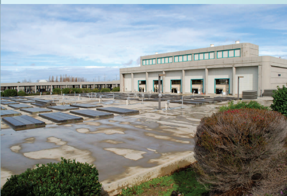
North City Water Reclamation Plant
