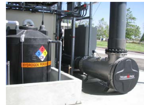
Advanced Oxidation with UV Light & Hydrogen Peroxide
