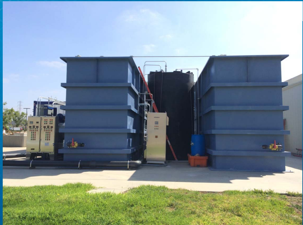
Biological Activated Carbon (BAC) Filters
