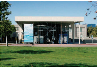
Advanced Water Purification Facility
