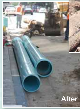
Cast iron water main replacement
