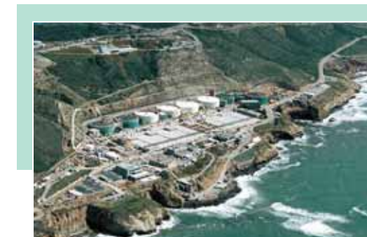
Point Loma Wastewater Treatment Plant
