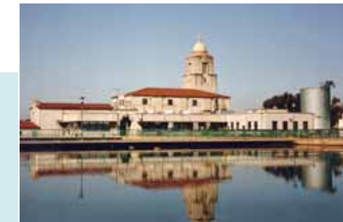
Alvarado Water Treatment Plant
