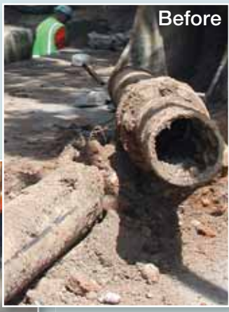
Cast iron water main replacement
