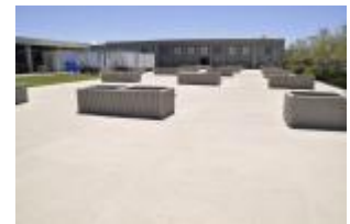
Chlorine contact basin where recycled water is treated with chlorine to kill any remaining bacteria.
