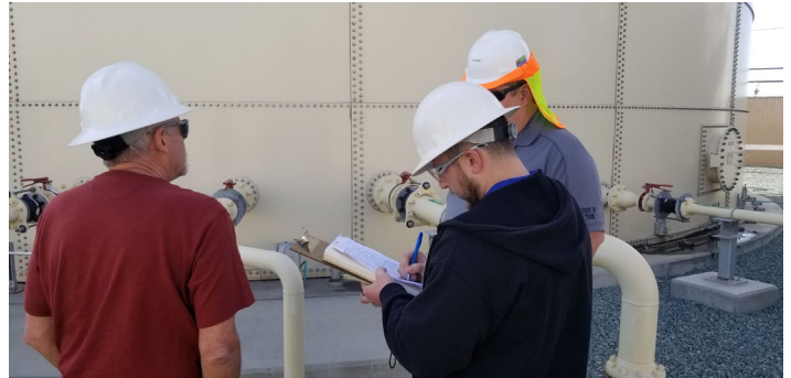
IWCP staff inspecting a water reclamation tank. Source: OCA.
