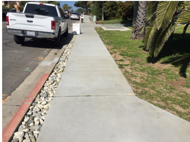
Original sidewalk (left) and improved sidewalk (right) with hydraulic disconnection
