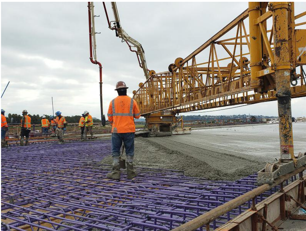
West Mission Bay Drive Bridge construction
