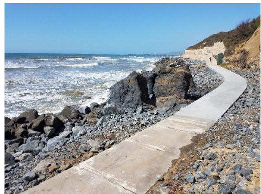
Orchard Ave walkway
