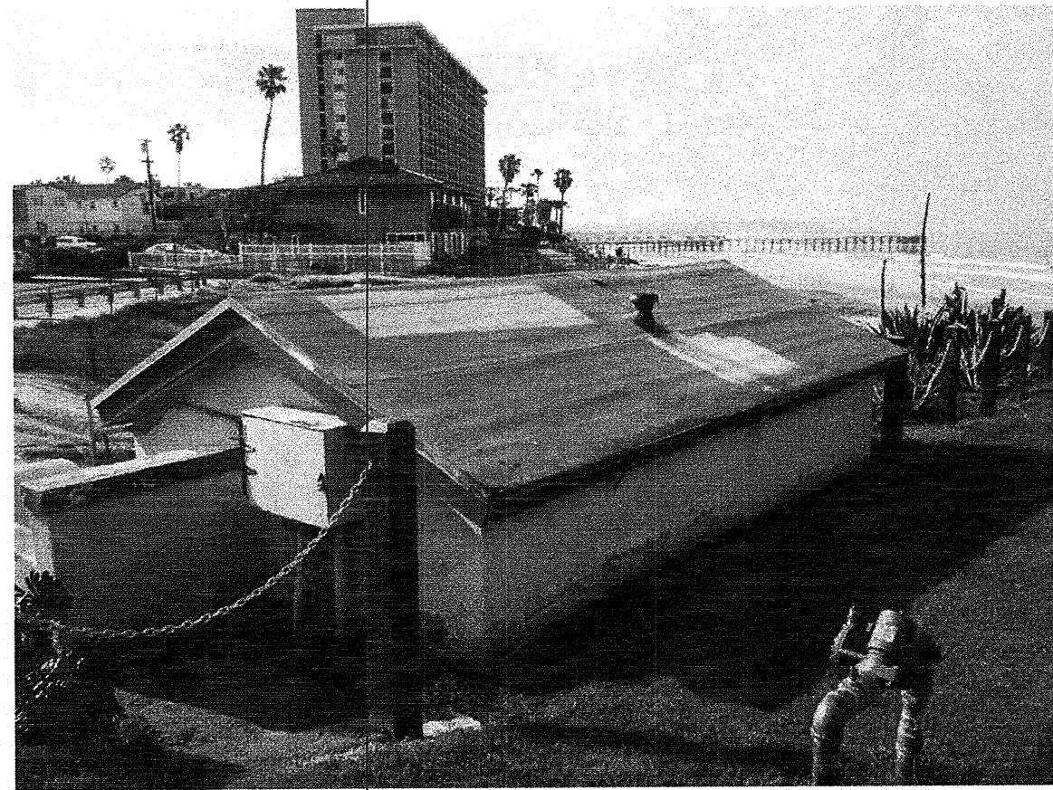
EXISTING PHOTO B
