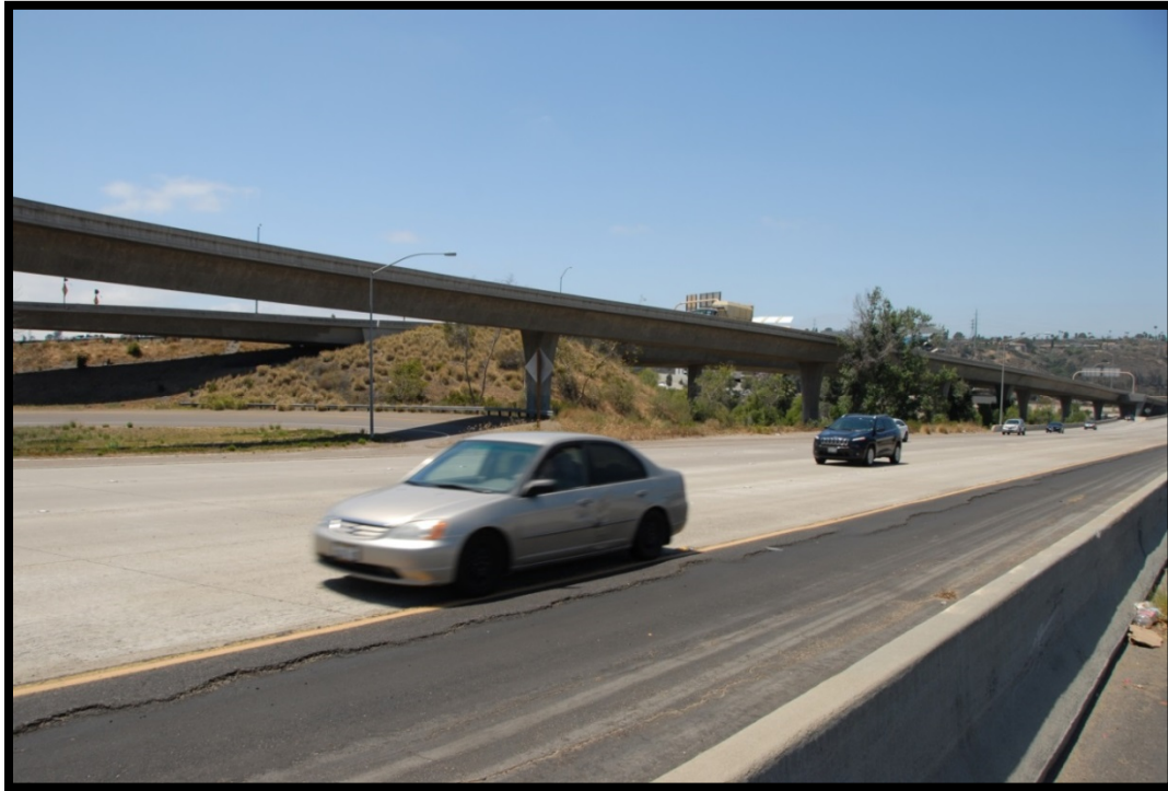
Figure 4.15-19 View 5—Northwestward View of Project from I-15
