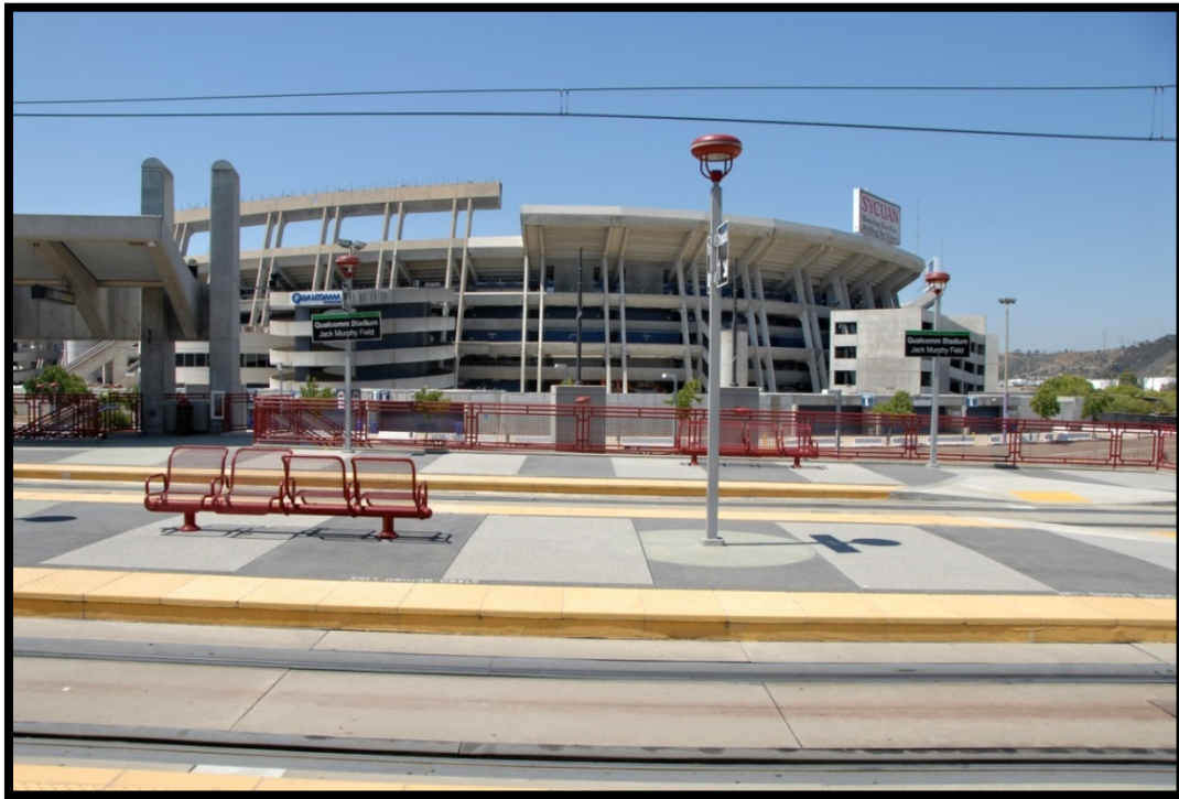
Figure 4.15-13 View 11—Northward View of Existing Project Site from MTS Stadium Station
