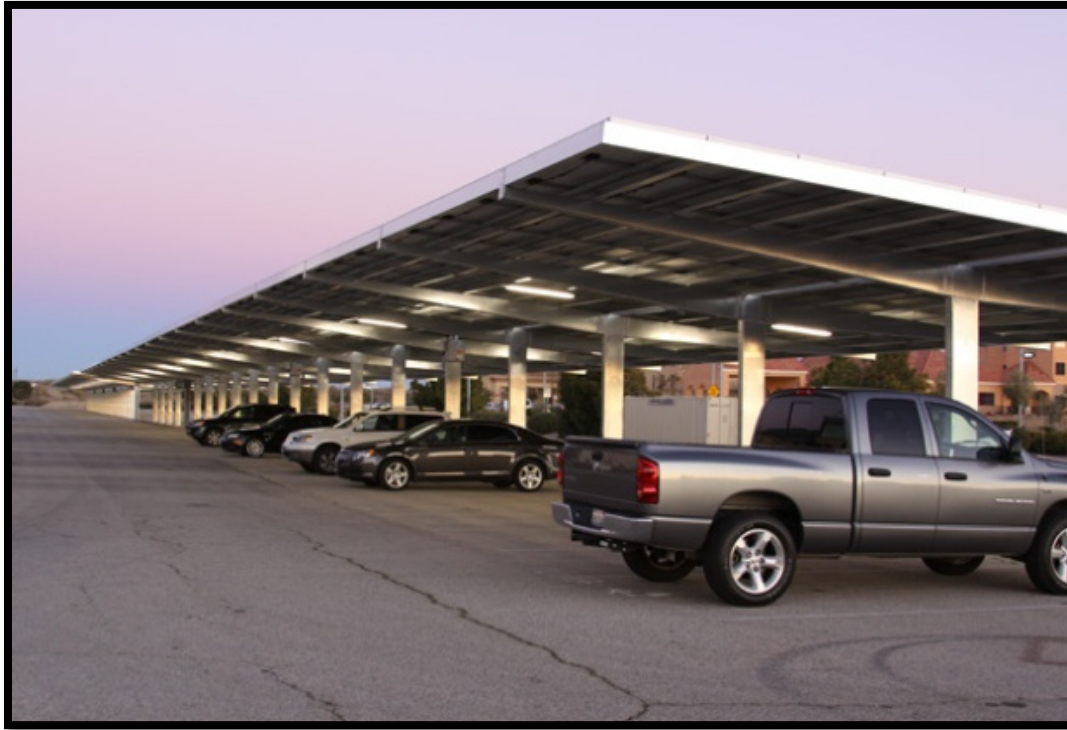
Figure 4.3-1. Typical T-Framed Solar Shade Canopy
