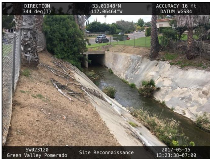
Figure 1: May 2017, looking downstream at double box culvert
