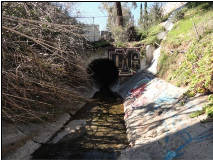
Figure 1: November 2016, facing downstream end of facility group; towards 60-inch-diameter RCP culvert beneath the Collwood Villas Apartments and Collwood Boulevard
