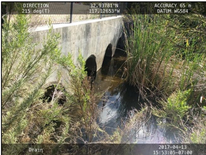
Figure 1: April 2017, looking upstream at quadruple-barrel 6-foot-diameter RCP storm drain outlet at Mercy Road
