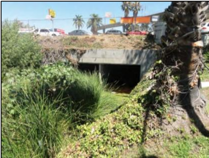
Figure 1: August 2014, looking upstream at the triple 12-foot-wide by 8-foot-tall RCB culvert beneath Fairmount Avenue
