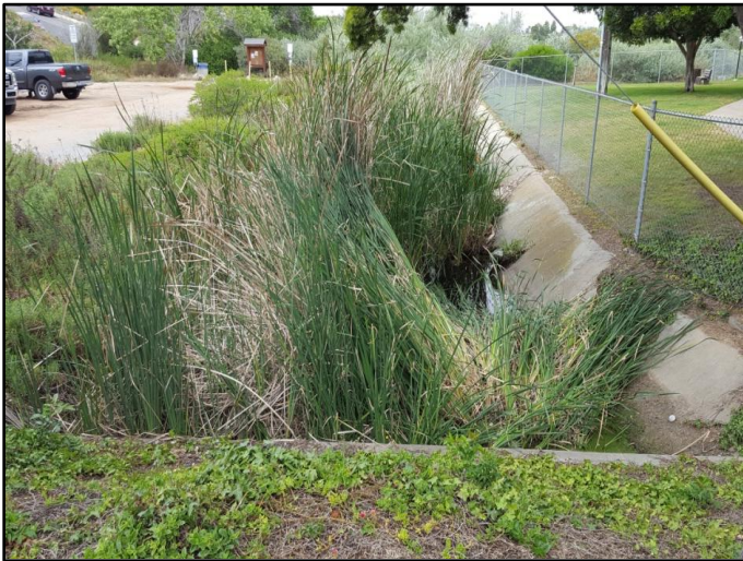
Figure 1: April 2017, looking downstream over headwall and 48-inch-diameter and 30-inch-diameter diameter RCP culvert outlet
