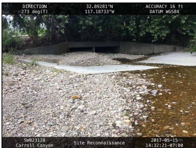
Figure 1: May 2017, sediment and cobbles accumulated on concrete inlet apron upstream of the culvert
