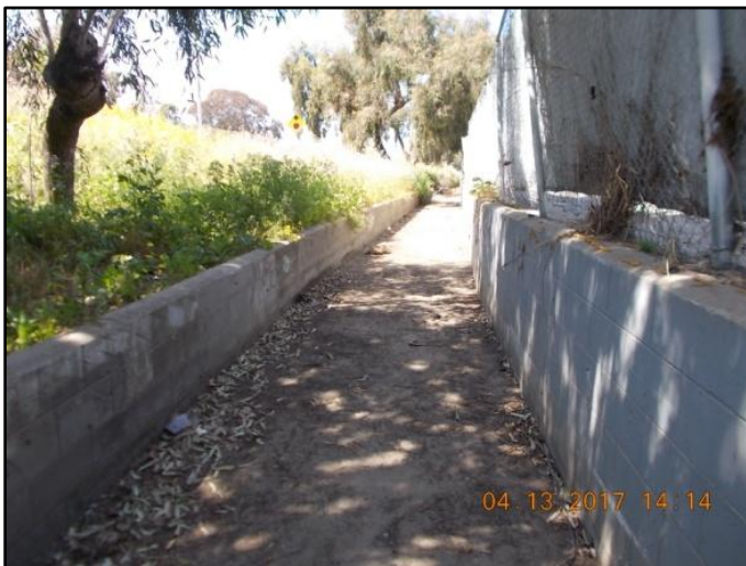
Figure 1: April 2017, looking downstream at sediment and debris at upstream end of concrete ditch
