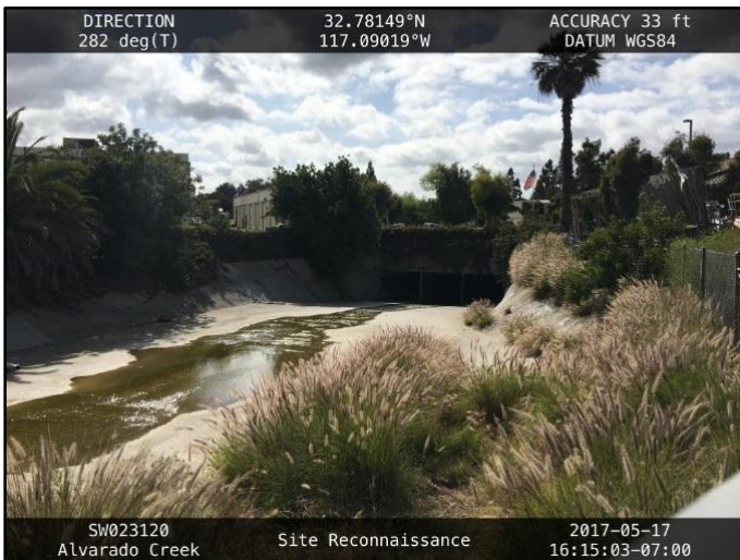
Figure 1: May 2017, looking at the downstream end of segment, towards the triple 9-foot wide by 8-foot high RCB culvert beneath Mission Gorge Place
