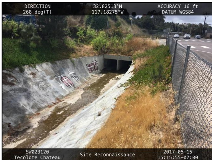
Figure 1: May 2017, upstream of double 5-foot-wide by 4-foot-high RCB culvert beneath Derrick Drive
