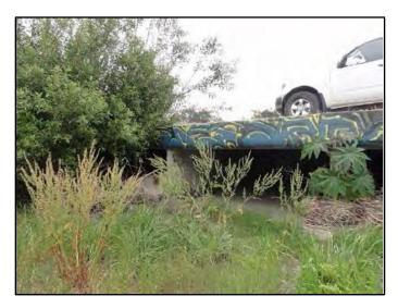
Figure 1: April 2015, looking downstream at entrance to quadruple 12-foot-wide by 4-foot-high RCB culvert beneath Interstate 5
