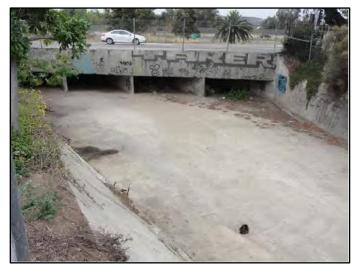
Figure 1: April 2015, looking downstream at entrance to quadruple 12-foot-wide by 4-foot-high RCB culvert beneath West San Ysidro Boulevard
