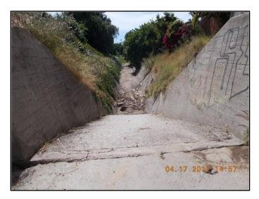
Figure 1: April 2017, looking downstream at second drop structure and sediment accumulated at bottom of structure
