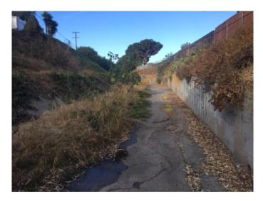
Figure 1: April 2017, looking downstream at accumulated sediment and debris in concrete channel
