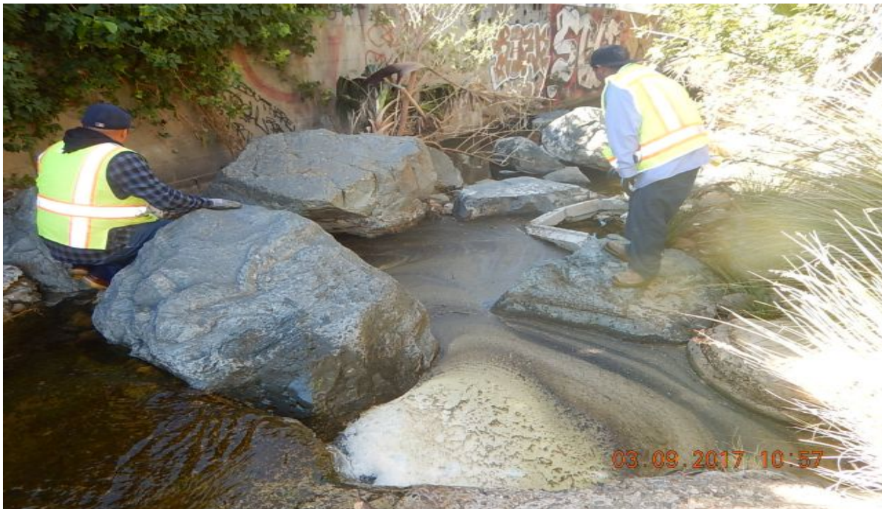
Upstream portion of South Chollas Creek Channel Map 101 Reach 2 facing south. This is the rip rap section of the channel, which marks the transitions from a concrete lined bottom to an earthen bottom.
