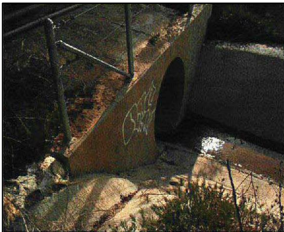
1. IHHA 1. Industrial 1, Reach 3: Looking at 54-inch-diameter RCP outlet at upstream end of facility group.
