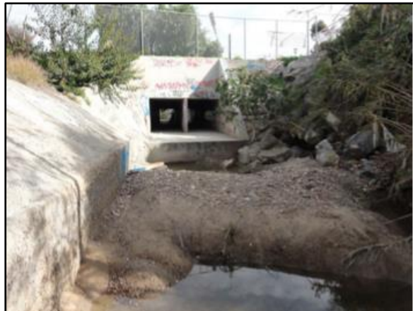
IHHA 10. Home 4, Map 1: Looking upstream at the double 6-foot wide by 6-foot tall RCB culvert. Note the standing water and erosion at culvert outlet.
