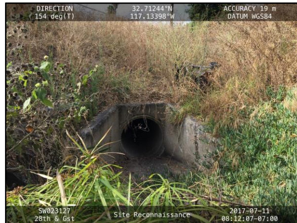
4. 28th St 1: 30-inch-diameter RCP culvert at downstream end of segment.
