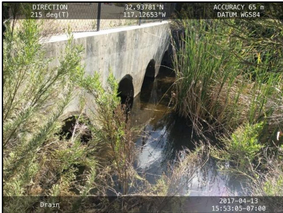
1. Black Mountain 2: Looking upstream at quadruple-barrel 72-inch-diameter RCP storm drain outlet at Mercy Road.
