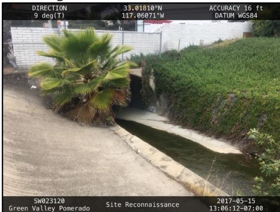
3. Pomerado 2: Looking downstream at CMP culvert at downstream end of segment.
