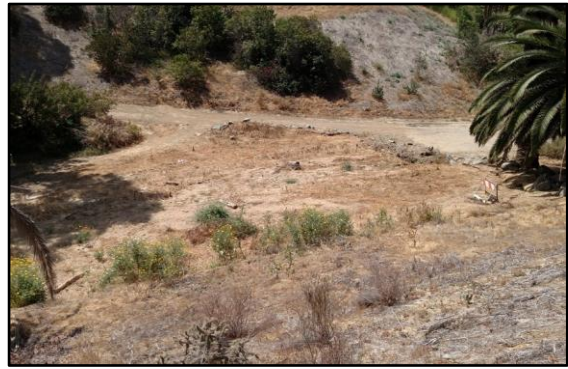
2. Maple Canyon: Looking south onto basin, completely filled with sediment.
