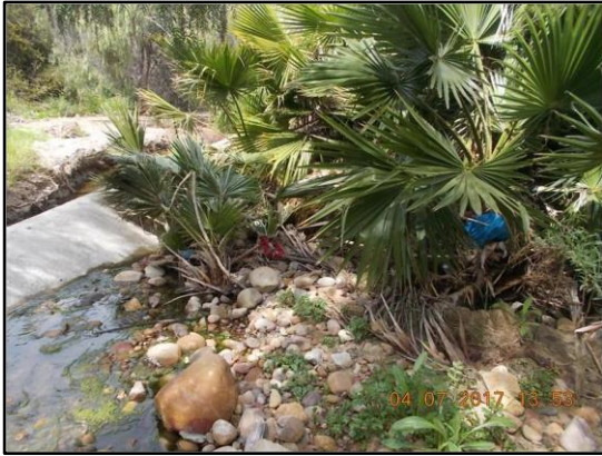
5. Fairmount 2: Looking downstream at sediment/debris and vegetation in concrete ditch.
