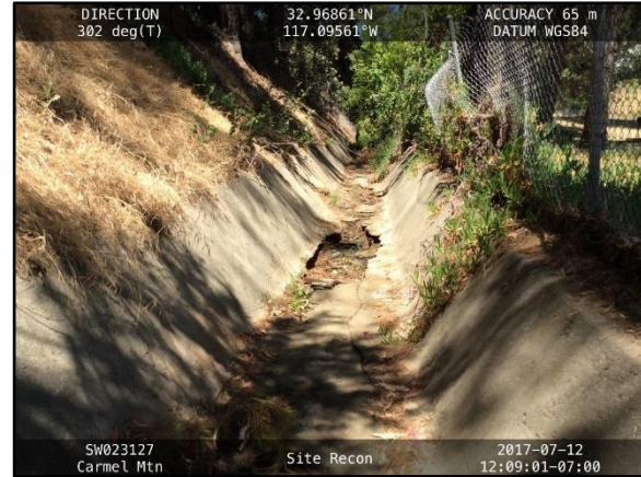
2. Via San Marco 1: Representative of segment showing failure of gunite bottom, looking upstream.
