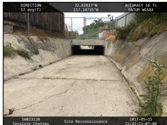
4. Chateau 2: Downstream of 10-foot-wide by 3-foot-high RCB culvert beneath Chateau Drive.
