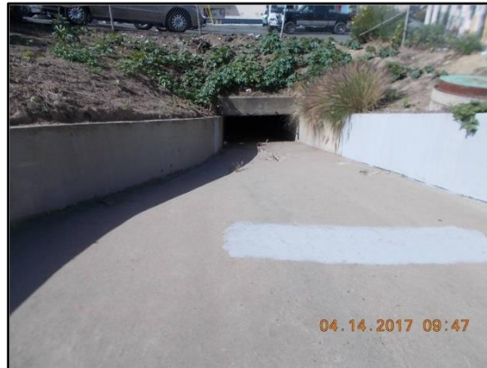
6. Downstream Domain of Analysis: Looking downstream at entrance to 2.5-foot by 6.5-foot RCB culvert inlet (April 2017).
