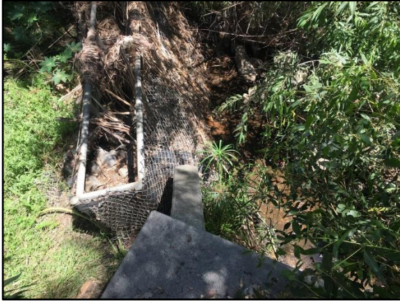
3. Paseo del Verano 1: Gabion wall structure at outlet structure.
