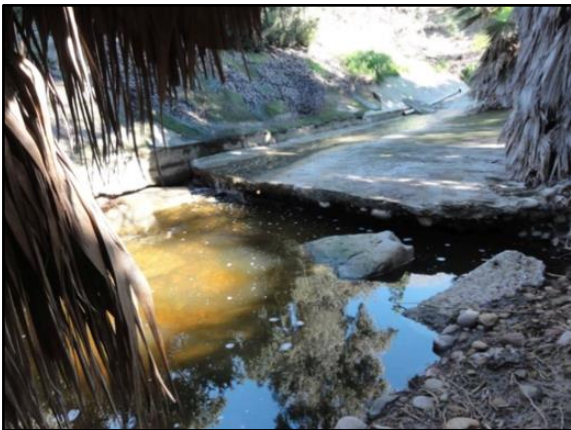
IHHA 9. Baja 1 (Reach 2): Facing the upstream end of Reach 2 towards transition from earthen bottomed to concrete lined immediately downstream of 60-inch-diameter RCP culvert beneath 54th Street.
