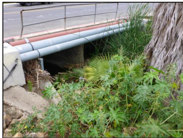
2. Rolando 2: Pre-maintenance; looking towards the double 8-foot wide by 5-foot, 2-inch tall RCB culvert at downstream end of segment.
