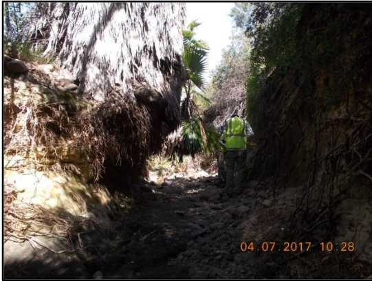
1. Aldine 1: Looking downstream at vegetation, erosion in facility.
