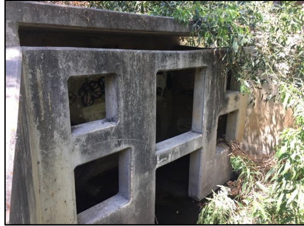
4. Paseo del Verano 1: Basin outlet structure.
