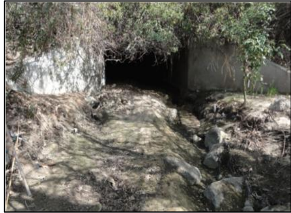
1. Home 1, Map 2: Looking the upstream end of the segment towards the 12-foot wide by 6-foot tall RCB culvert under Terrace View Villas.
