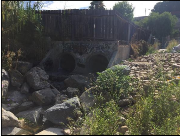
3. Wightman 2: Looking upstream at double 42-inch-diameter RCP; split flow into parking lot seen to the left.
