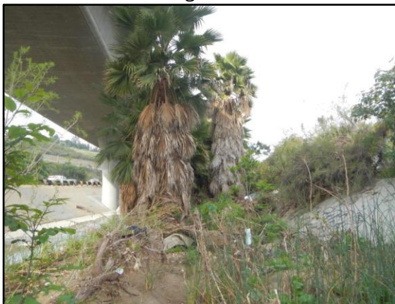
5. Mission Gorge 3, Map 1 (March 2019), Looking downstream adjacent to the overpass. Sediment accumulation, palms, and vegetation evident on right half of channel, left half (lined) is mostly clear).
