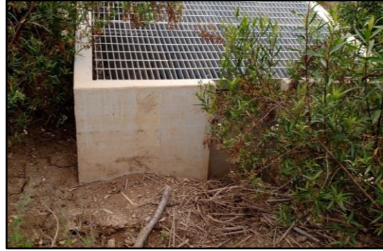
4. Alta La Jolla: Outlet structure observed to be partially blocked with sediment/debris.
