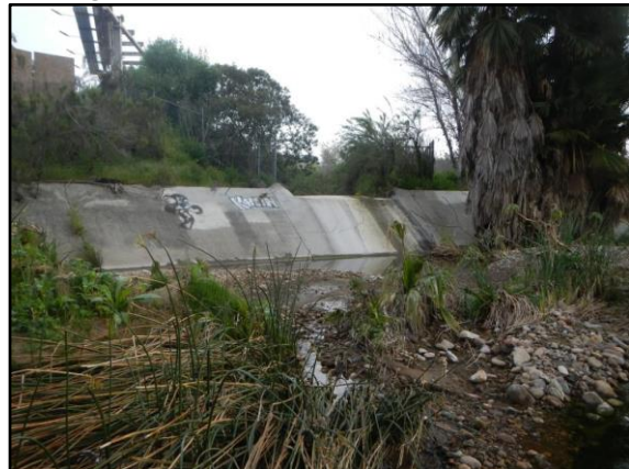
4. Mission Gorge 3, Map 1 (March 2019), Looking north at scour hole at outlet of tributary channel.
