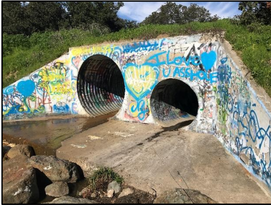
1. Genesee1: Looking upstream at dual 84-inch-diameter and 54-inch-diameter CMP culvert outlet.
