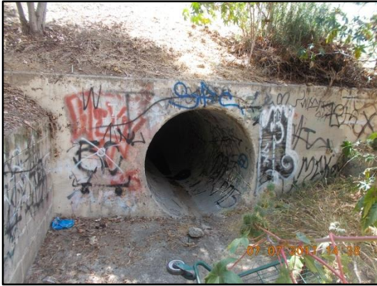
3. Martin 1: Looking downstream at 60-inch-diameter RCP culvert entrance under 35th Street.
