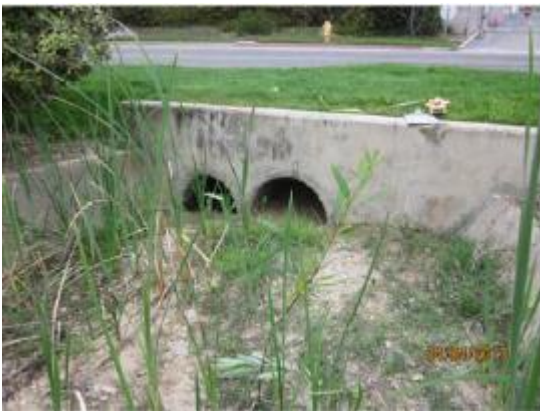
IHHA 62. Flintkote 1: Looking upstream at the 24- and 30-inch RCP outlet.
