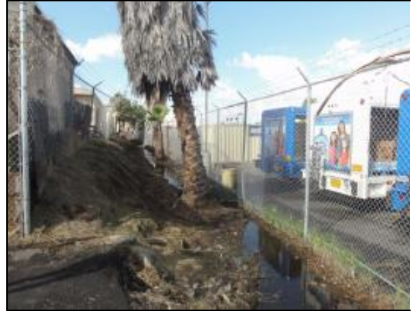
IHHA 15. Engineer 1 (Reach 2): Upstream portion of reach facing west, showing sediment and vegetation in ditch (November 2015).
