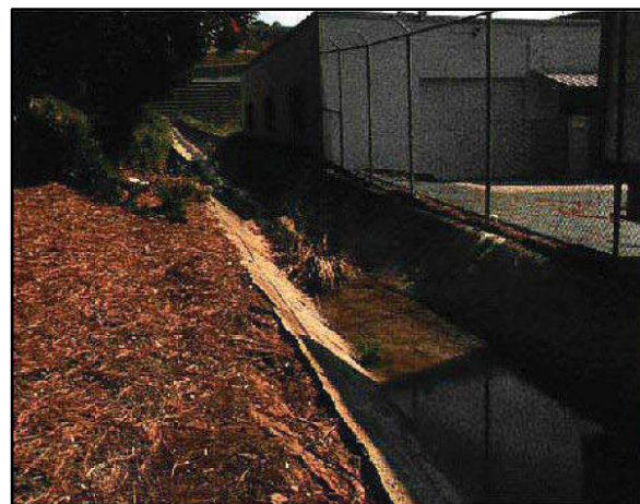
2. IHHA 4. Industrial 1, Reach 3: Looking upstream at minor vegetation and sediment within concrete segment.
