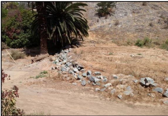
3. Maple Canyon: Basin completely filled with sediment.
