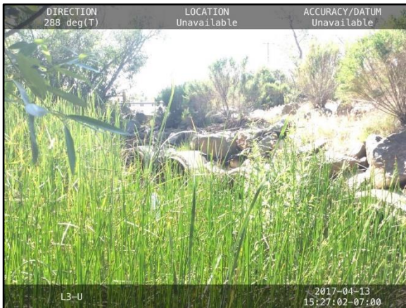
3. Black Mountain 2: Looking downstream at the seven-barrel 54-inch-diameter RCP culvert beneath the Canyonside Ranch driveway.
