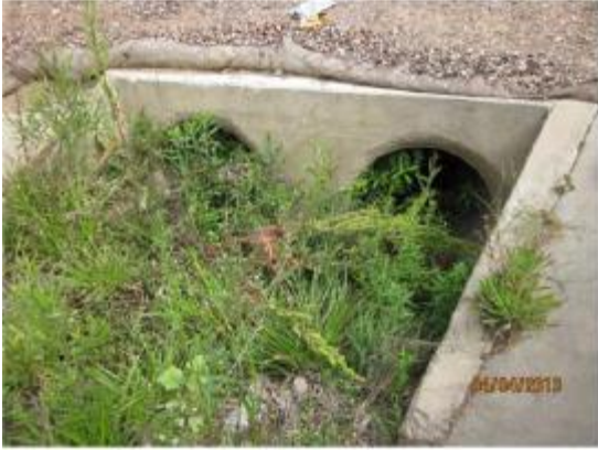
IHHA 79. Flintkote 1: Looking downstream at the double-barrel 36-inch RCP culvert entrance at downstream end of facility group.
