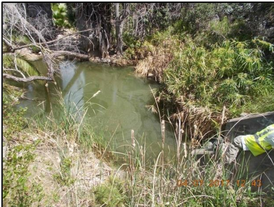
3. Fairmount 3: Looking downstream at scour pool at channel outfall.
