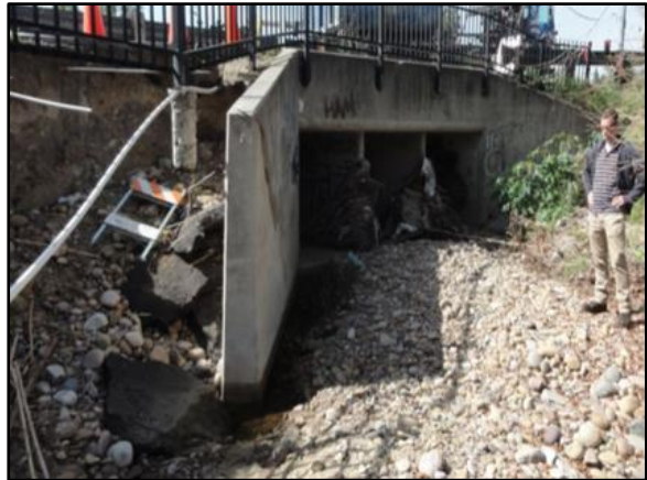
3. Home 1, Map 2: Standing along east bank of segment, looking southwest at erosion behind east wing wall at downstream end.
