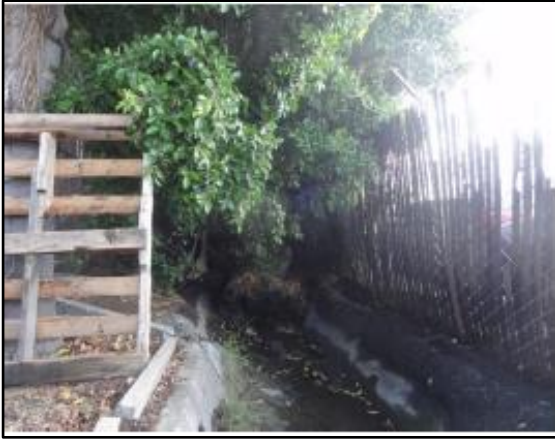
IHHA 8. Engineer 1 (Reach 2): Downstream portion of reach facing east at vegetation blocking the ditch (November 2015).
