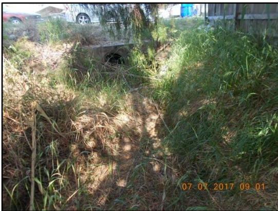
5. J St 1 (Reach 1): Looking downstream at 30-inch-diameter RCP culvert inlet on east side of Toyne Street
