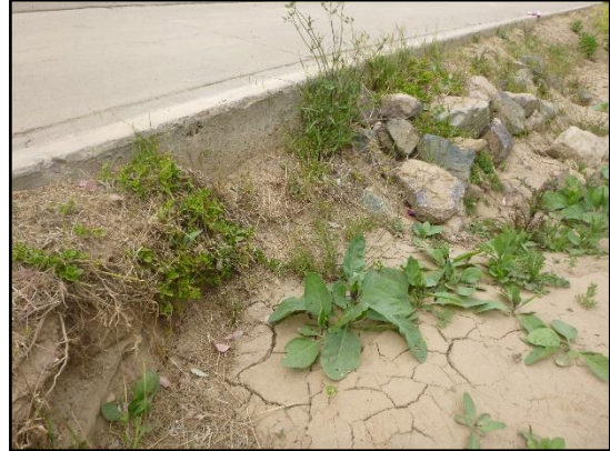
1b. Dunhill 1: Looking at bank erosion along Dunhill Street.
