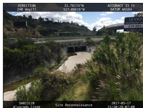
2. Mission Gorge 4, Map 1: Looking downstream at the triple 9-foot-wide by 8-foot- wide.
