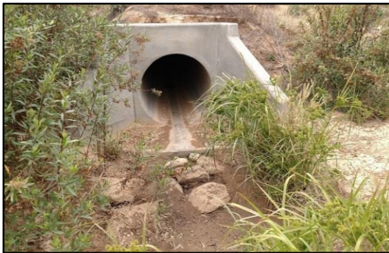
1. Alta La Jolla: Inlet observed to be mostly clear of sediment/debris.
