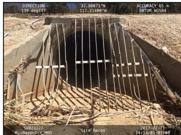
4. Mission Bay Drive 1: Recently maintained culvert inlet at downstream end of segment.
