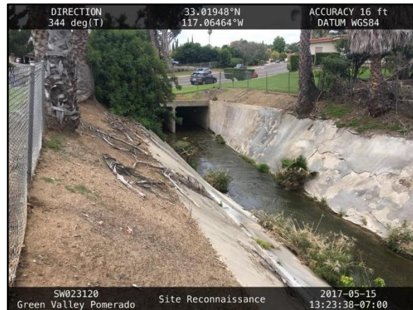
4. Pomerado 1: Looking downstream at double box culvert.
