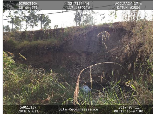
2. 28th St 1: Eroded eastern sidewall.
