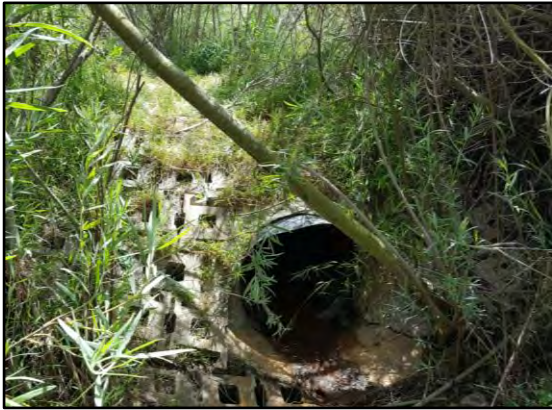
5. Downstream Domain of Analysis: Looking upstream at 24-inch-diameter PVC culvert through pedestrian trail.
