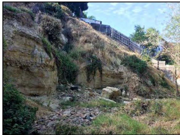
2. Wightman 2: Looking downstream toward channel bank failure/erosion.
