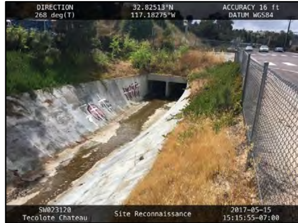
2. Chateau 1: Upstream of double 5-foot-wide by 4-foot-high RCB culvert beneath Derrick Drive.
