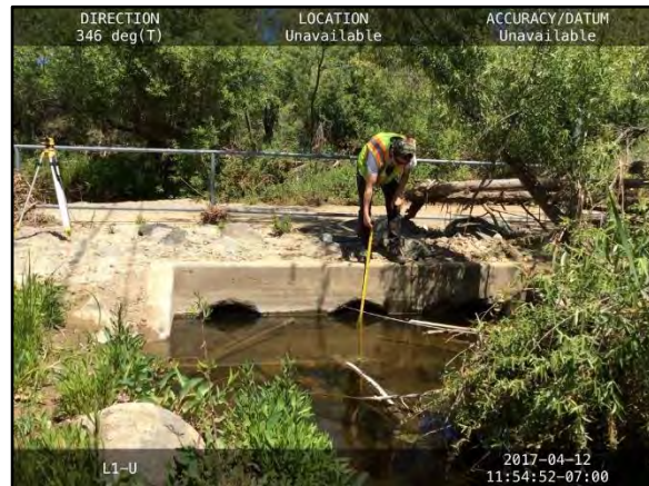
4. Black Mountain 2: Looking downstream at triple barrel 24-inch-diameter RCP beneath the Los Peñasquitos Canyon Trail.
