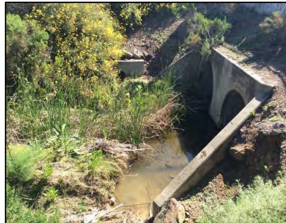
4. Black Mountain 1: Looking downstream at the double barrel 72-inch-diameter RCP culvert.
