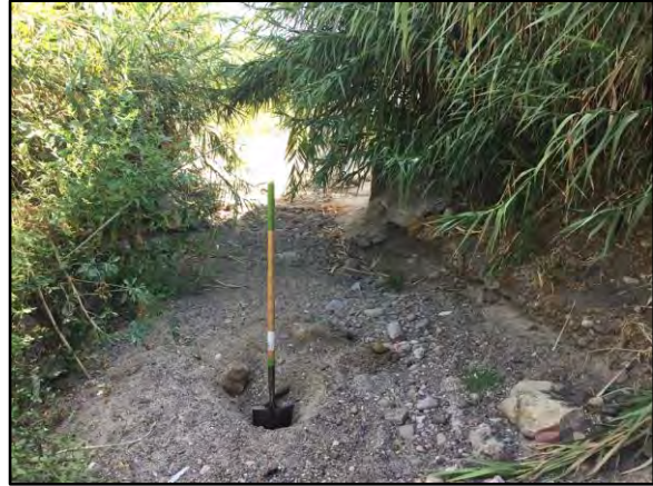
4. Wightman 1: Looking upstream just after transition from concrete to earthen lining; deep sediment observed.
