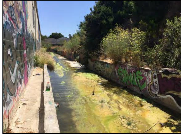
4. Cartagena 1: Looking upstream; missing sidewall and eroded bank at center.
