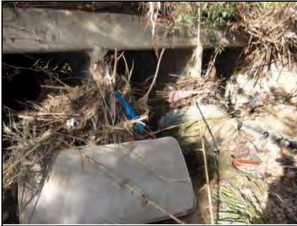
IHHA 1. Home 2, Map 1: Looking downstream at the triple 6-foot wide by 6-foot tall RCB culvert under Spillman Drive. Photo shows 50% clogging of culvert.
