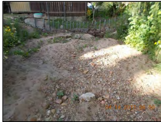
4. Titus 1: Looking downstream at sediment/debris accumulated at debris fence.
