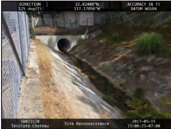
1. Chateau 1: Downstream of 72-inch-diameter CMP culvert beneath Chateau Drive at Paola Way.
