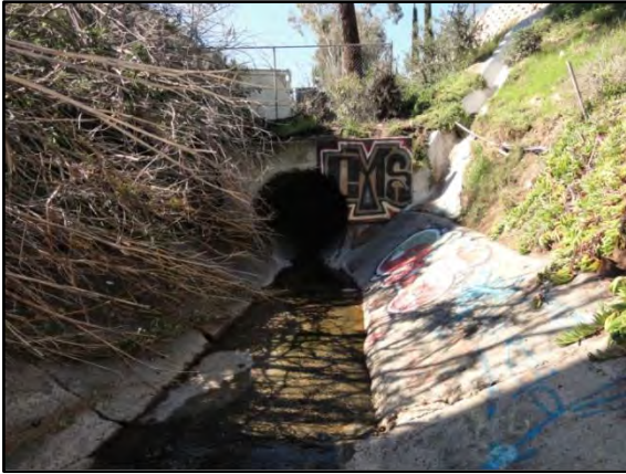
IHHA 1. Baja 1 (Reach 1): Facing downstream end of facility group; towards 60-inch-diameter RCP culvert beneath the Collwood Villas Apartments and Collwood Boulevard.
