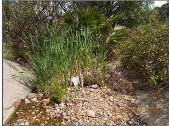
2. Fairmount 4: Looking downstream at sediment/debris and vegetation in concrete ditch.
