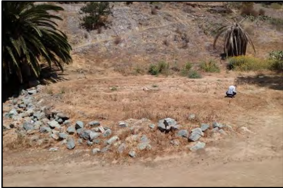
1. Maple Canyon: Sediment deposition observed in basin and minimal vegetation growth within basin.
