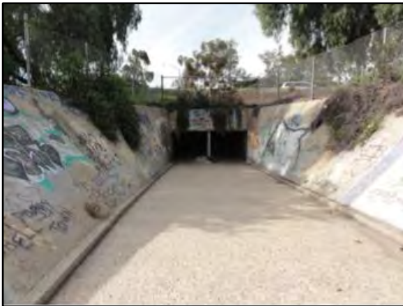
IHHA 6. Home 3, Map 1: Looking downstream towards 7-foot wide by 6-foot tall double RCB culvert. Note clean channel.
