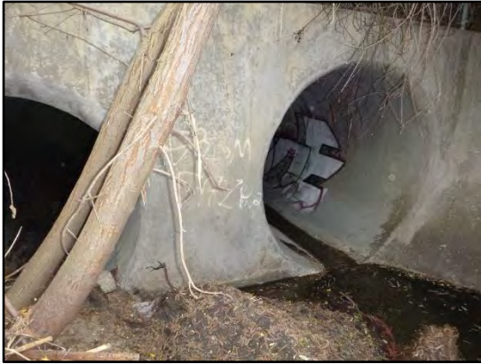
5. Genesee 1: Looking downstream at dual 84-inch-diameter and 72-inch-diameter RCP culvert inlet.
