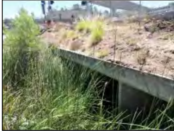
IHHA 5. Mission Gorge 1, Map 2: Looking at downstream end towards the triple 8-foot-wide by 12-foot-tall RCB culvert beneath Fairmount Avenue.
