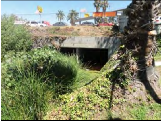
IHHA 3. Mission Gorge 1, Map 2: Looking upstream at the triple 8-foot-wide by 12-foot-tall RCB culvert beneath Fairmount Avenue.
