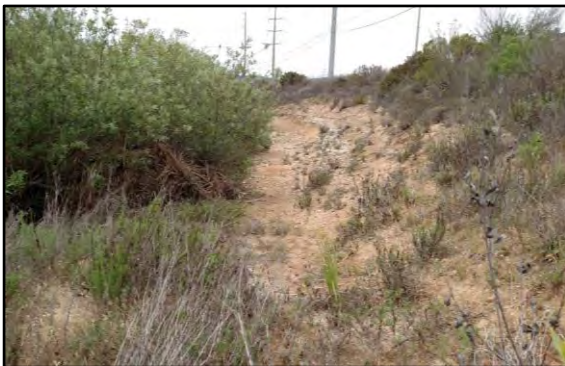
1. 5-805 Basin: Looking downstream at heavily vegetated inlet to basin from upstream end.
