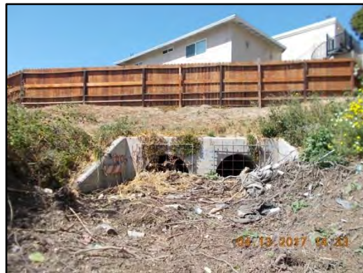
6. Nimitz 1: Looking downstream at dual 54-inch diameter RCP culvert inlet.
