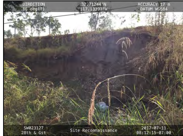
2. 28th St 1: Eroded eastern sidewall.
