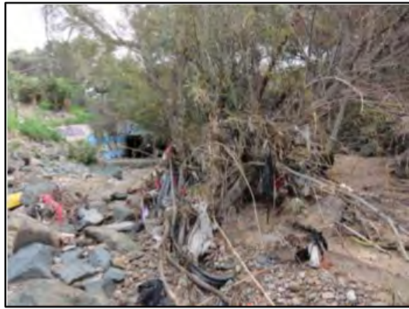
IHHA 4. Home 2, Map 1: Looking upstream at the vegetation and displaced riprap downstream of the double 7-foot wide by 6-foot tall RCB culvert.
