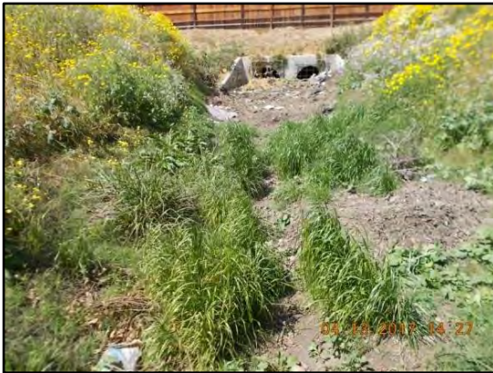
5. Nimitz 1: Looking downstream at sediment/debris in segment and at entrance to dual 54-inch diameter RCP culvert inlet.
