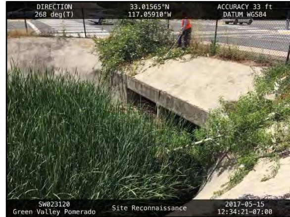
2. Pomerado 2: Looking downstream at double box culvert.
