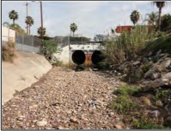
IHHA 13. Home 5, Map 1: Looking upstream at the double-barrel 74-inch-diameter RCP culvert.
