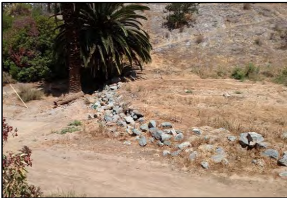
3. Maple Canyon: Basin completely filled with sediment.
