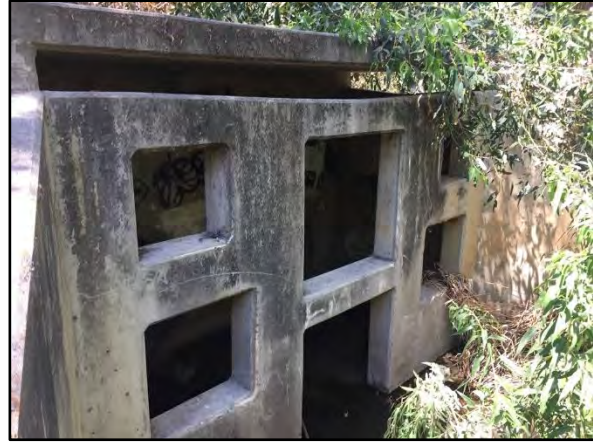
4. Paseo del Verano 1: Basin outlet structure.
