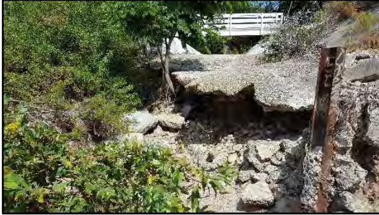
7. Megan 1, Reach 1: Looking upstream at erosion under concrete bottom at ditch outfall to Chollas Creek.
