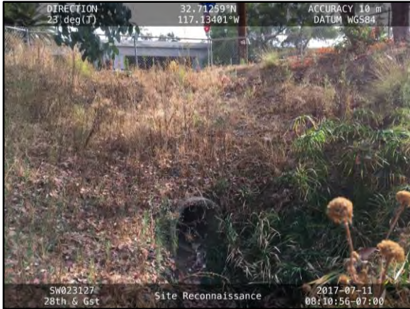
1. 28th St 1: RCP culvert outlet at upstream end of segment.
