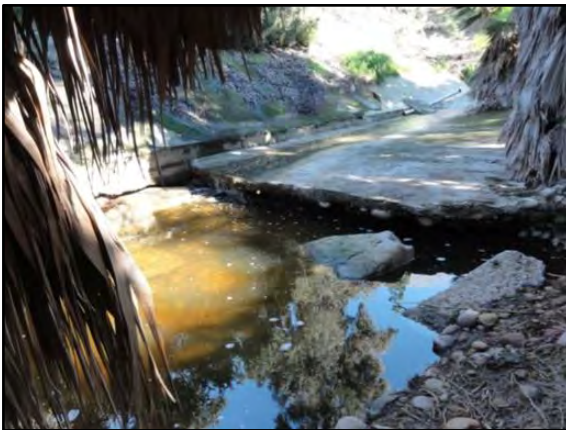
IHHA 9. Baja 1 (Reach 2): Facing the upstream end of Reach 2 towards transition from earthen bottomed to concrete lined immediately downstream of 60-inch-diameter RCP culvert beneath 54th Street.
