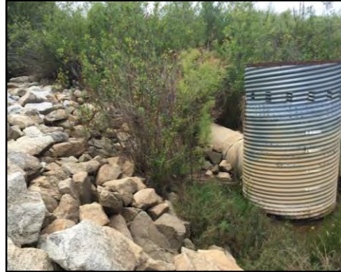
4. 5-805 Basin: Basin outlet structure and rip rap embankment.
