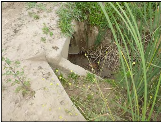
6. Dunhill 1: Looking downstream at entrance to 54-inch-diameter RCP culvert inlet.
