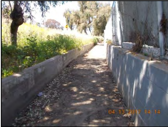
3. Nimitz 2: Looking downstream at debris/sediment at upstream end of concrete ditch.
