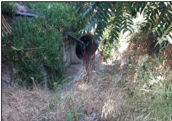
1. Jamacha 3: Looking upstream from Beacon Drive culvert (36-inch-diameter RCP).
