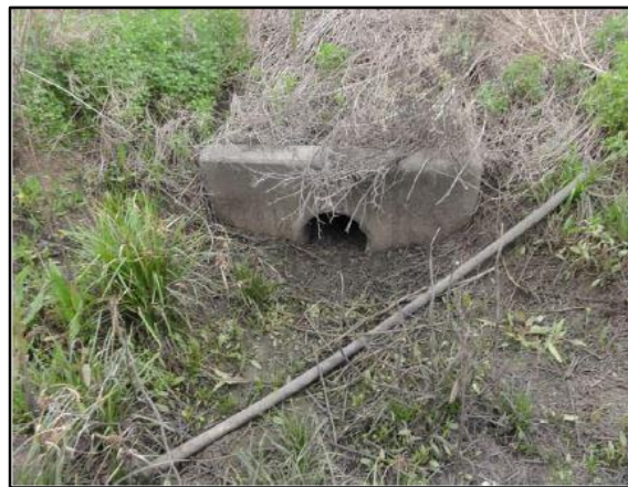
IHHA 22. Detention Basins: 18-inch-diameter RCP connecting the two detentions basins in the shared detention facility.
