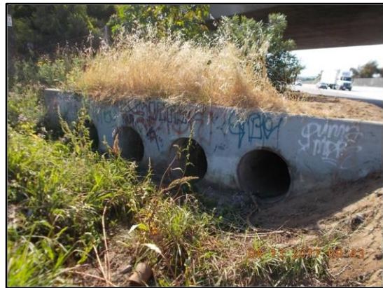
6. Outer 1, Reach 1: Looking downstream at entrance to quadruple 30-inch-diameter RCP culvert inlet.
