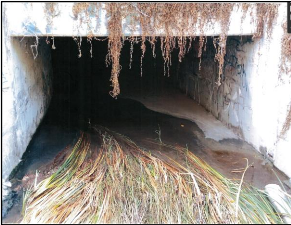
4. Via de La Bandola 11, Map 1: 8-foot-wide by 4-foot-high RCB culvert at downstream end of channel (Station 1418); no observed sediment or vegetation in culvert.
