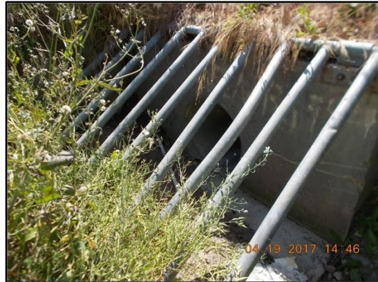
4. Castana 1: Looking downstream at 24-inch-diameter RCP culvert inlet.
