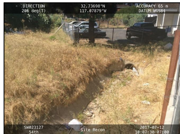
2. 54th St 1: Looking downstream towards the culvert; conveys flows beneath parking lot, then discharges back into ditch.
