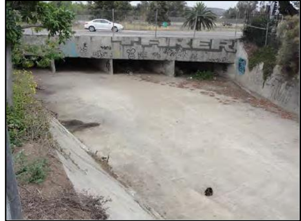
IHHA 11. Via Encantadoras 2, Map 2 (Reach 1): Looking downstream at entrance to quadruple 12-foot-wide by 4-foot-high RCB culvert beneath West San Ysidro Boulevard.
