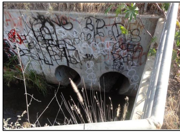
IHHA 24. 30 th St 1: Looking downstream at the double-barrel 36-inch-diameter RCP culvert at the San Diego Railroad crossing (May 2015).
