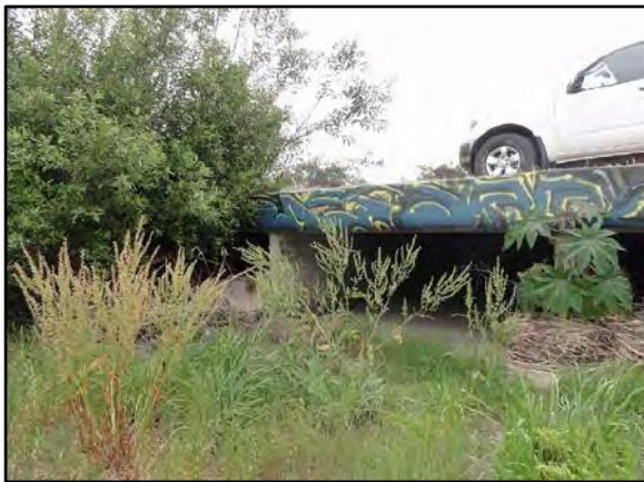
IHHA 14. Via Encantadoras 1, Map 2 (Reach 1): Looking downstream at entrance to quadruple 12-foot-wide by 4-foot-high RCB culvert beneath Interstate 5.
