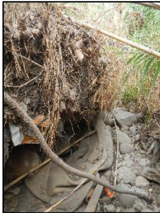
9. Lobrico 1, Reach 1: Second head cut erosion along bottom of channel, measuring 2 feet in height, looking southwest (July 2019).
