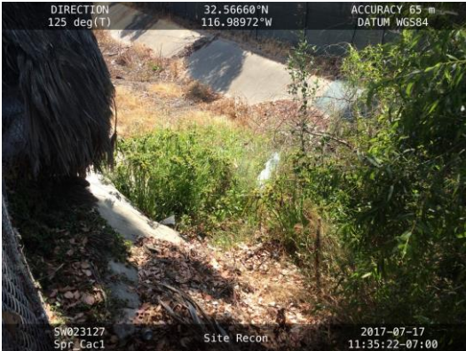
1. Cactus 2: Sediment deposition and vegetation growth at inlet.
