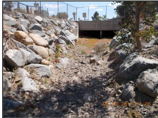
6. Tocayo 1: Looking upstream vegetation and outlet of double 10-foot by 4-foot RCB culvert.
