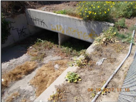
5. Tocayo 2: Looking downstream at inlet to double 10-foot by 4-foot RCB culvert.
