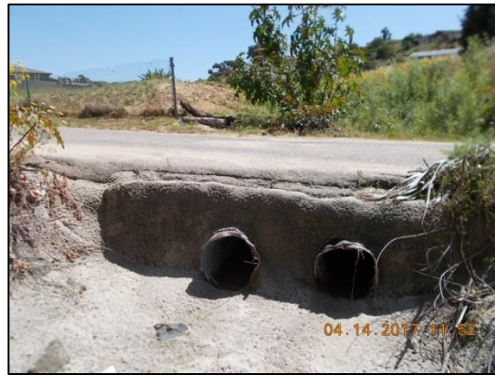
2. Cervantes 1: Looking upstream at double 18-inch-diameter CMP culvert and Arizona crossing at Cervantes Road.
