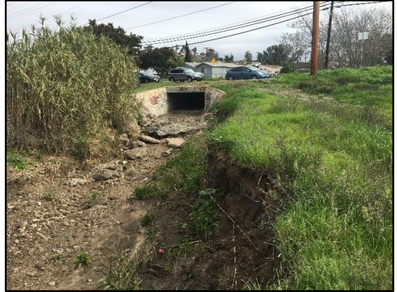
4. Jamacha 1: Upstream of 10-foot-wide by 5-foot-high RCB culvert beneath 69th Street facing west.
