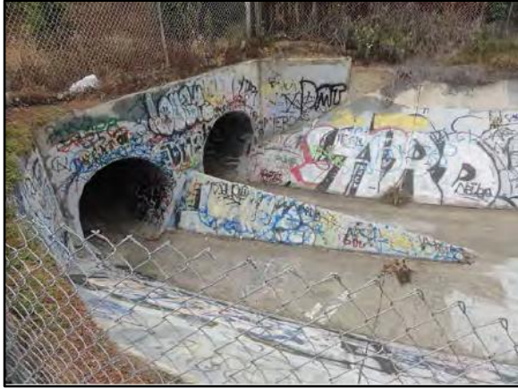
IHHA 9. Via Encantadoras 3, Map 2 (Reach 2): Entrance to double-barrel 72-inch-diameter RCP culvert under Vista Lane.
