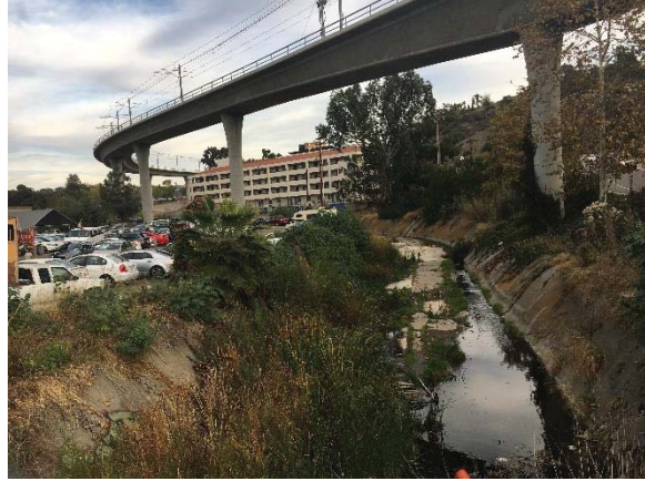
Looking upstream from Fairmount Avenue at approximately Station 1305.414 (November 2018).
