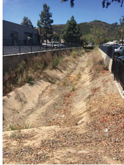
Looking upstream from approximately Station 49.81 (June 2018).
