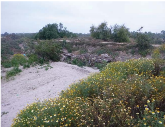
Looking at the culvert inlet at approximately Station 2549.85 (May 2017).
