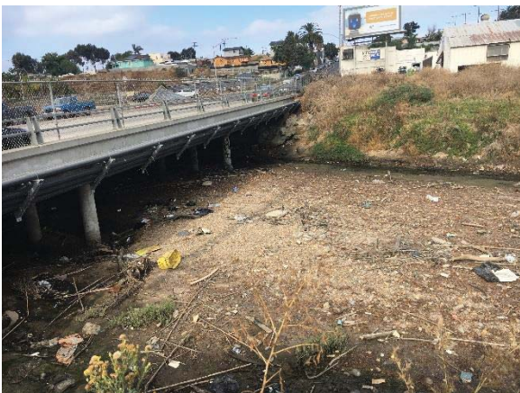
Looking downstream toward the National Avenue bridge at approximately Station 1745.9117 (August 2019).
