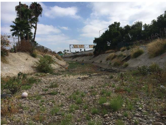
Looking upstream from approximately Station 2065.8479 (August 2019).
