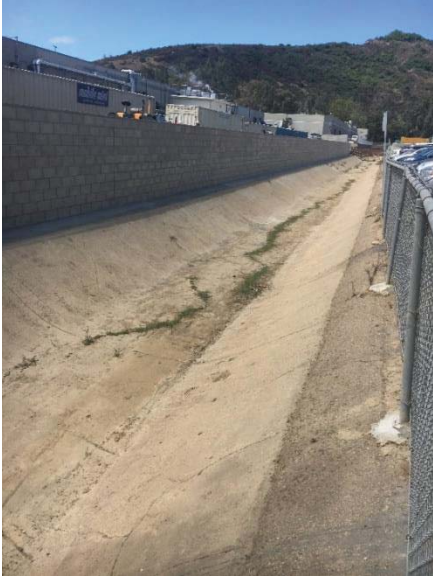
Looking upstream from approximately Station 400.82 (June 2018).
