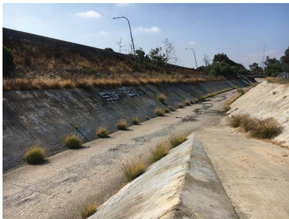
Looking downstream from approximately Station 4774.1509 (August 2019).
