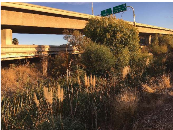
Looking downstream from Station 628.163 (June 2018).
