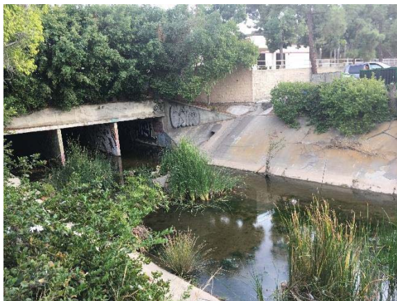
Looking upstream at the box culvert outlet at approximately Station 3519.105 (November 2018).
