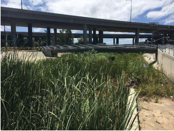
Looking upstream from approximately Station 3930.989 (June 2018).
