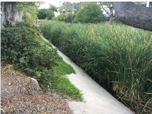
Looking upstream from approximately Station 3171.452 (November 2018).
