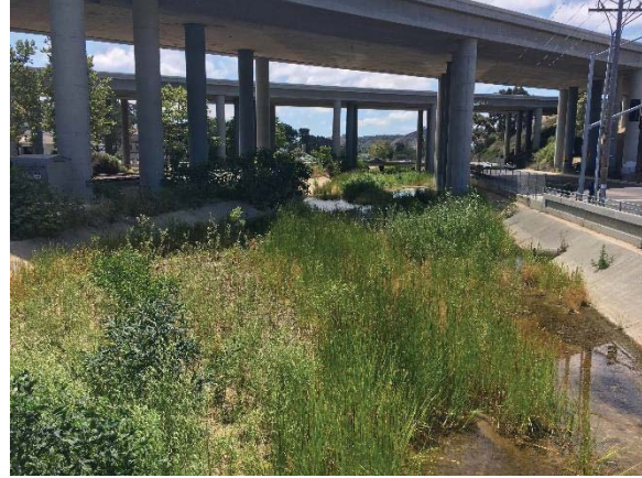
Looking upstream from approximately Station 4067.9646 (June 2018).
