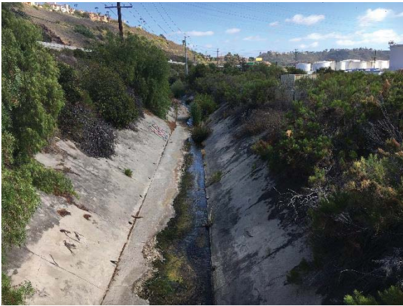
Looking upstream from approximately Station 530.489 (June 2018).
