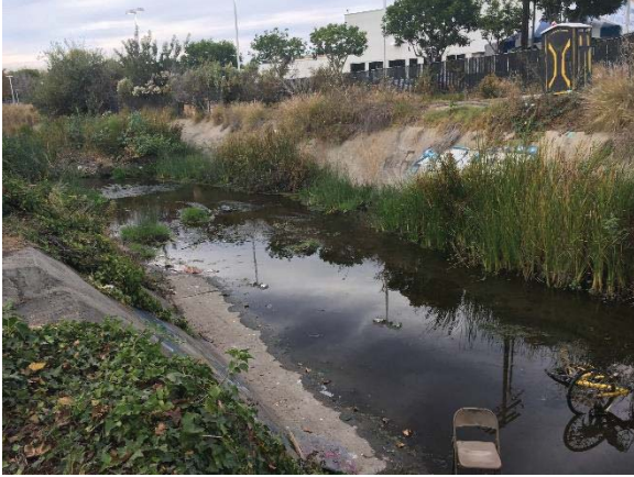
Looking downstream from the Fairmount Avenue culvert outlet at approximately Station 1155.562 (November 2018).
