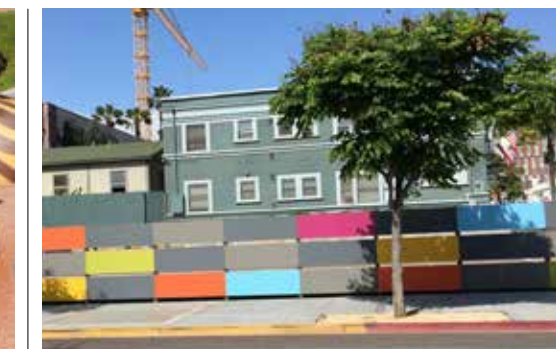
Railings and Fencing
