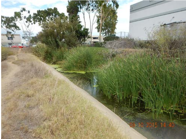
Nestor Creek Channel with vegetation and ponded water observed. Facing southeast in open field near 30 th Street.
