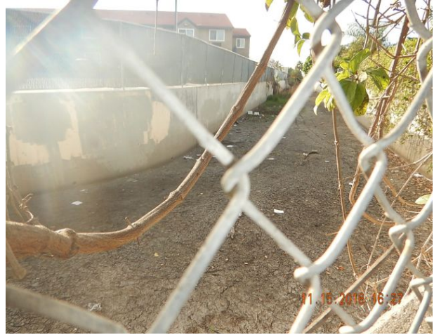
Nestor Creek Channel with vegetation and debris observed. No water observed in channel. Facing west along Reach 1b.
