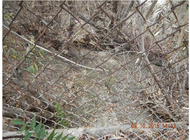
Nestor Creek Channel with vegetation and no dry weather flow observed. Facing east from 25 th Street near Grove Avenue.
