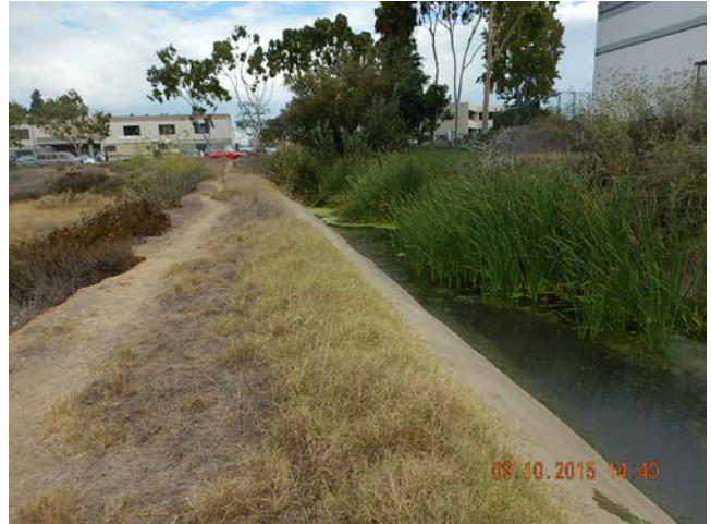
Nestor Creek Channel with vegetation and ponded water observed. Facing east on north edge of channel in open field near 30 th Street.
