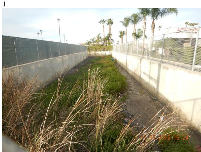
Nestor Creek Channel with vegetation and debris observed. No water observed in channel. Facing north along Palm Avenue.
