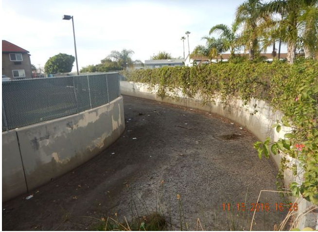
Nestor Creek Channel with debris observed. No water observed in channel. Facing northwest along Reach 1b.
