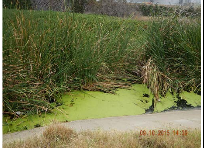
Nestor Creek Channel with vegetation and ponded water observed. Facing south in open field near 30 th Street.
