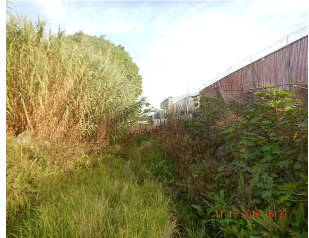
Nestor Creek Channel with dense vegetation observed. No water observed in channel. Facing east on northwest edge of channel in open field at the downstream end of Reach 1a.
