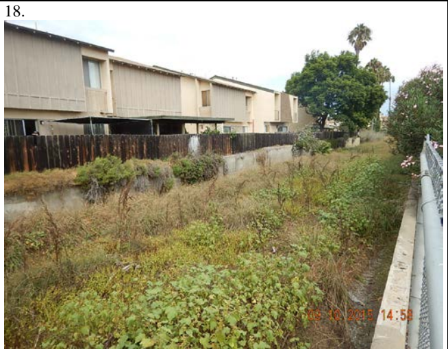
Nestor Creek Channel with vegetation and no dry weather flow observed.
