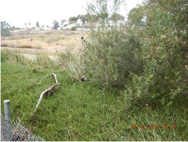
Nestor Creek Channel with vegetation and ponded water observed. Facing northwest near 30 th Street.
