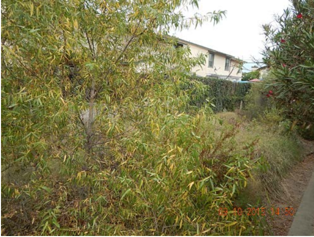
Nestor Creek Channel with vegetation and no dry weather flow observed. Facing northeast from south edge of channel along Grove Avenue near 27 th Street.
