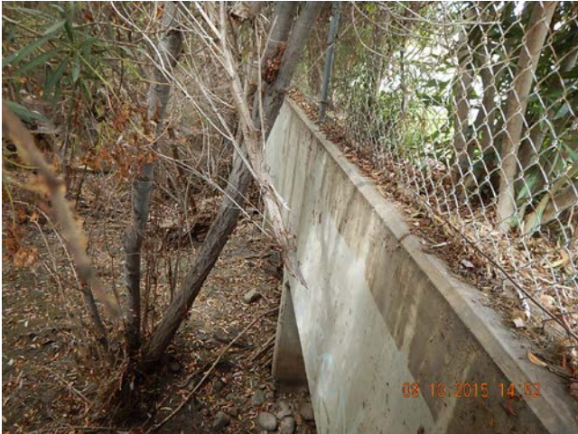
Nestor Creek Channel with vegetation and no dry weather flow observed. Facing south from 25 th Street near Grove Avenue.
