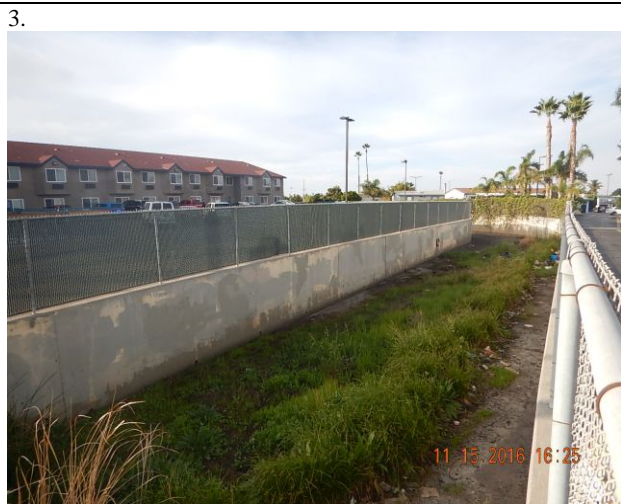
Nestor Creek Channel with vegetation and debris observed. No water observed in channel. Facing northwest along Reach 1b.
