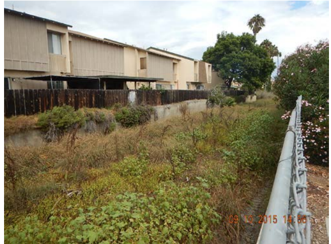
Nestor Creek Channel with vegetation and no dry weather flow observed.
