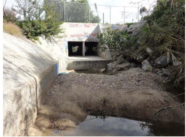
Upstream end of Reach 4 viewing north-east (upstream) at the 6 ft. by 6 ft. double box culvert. Note erosion at culvert apron.
