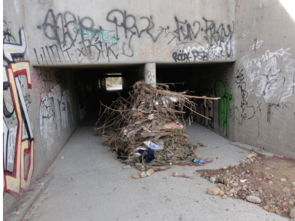
Reach 5 viewing south-west (downstream) at the 6 ft. by 6 ft. double box culvert.
