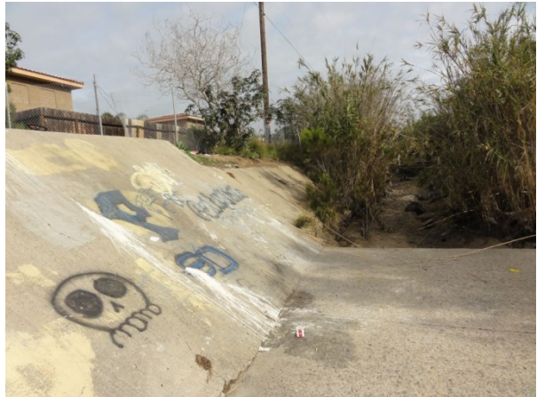
Connection of Reach 3 and Reach 4 where channel changes from concrete lined, to earthen bottom and earthen southeast sideslope. Viewing north-east (upstream).
