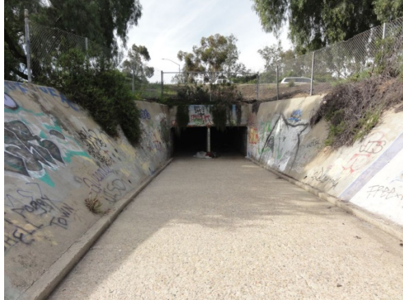
Downstream portion of Reach 3 viewing south-west at 7 ft. by 6 ft. double box culvert. Note clean channel.
