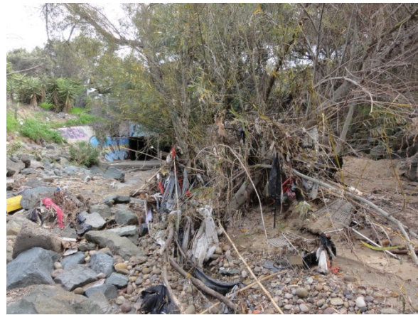
Upstream portion of Reach 2 viewing north-east (upstream) at the vegetation and displaced rip rap downstream of the double 7-ft. by 6-ft. double box culvert.
