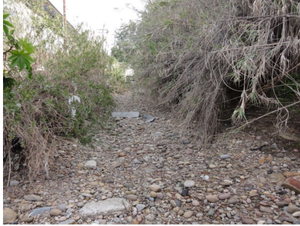
Reach 4 viewing north-east (upstream) at the vegetation compromising northwest concrete side slope
