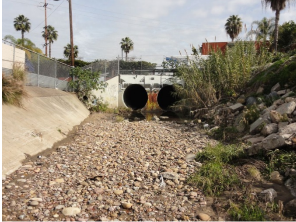
Upstream portion of Reach 5 viewing north-east (upstream) at the 74" double concrete pipe culvert. Note the standing water and erosion at culvert outlet.
