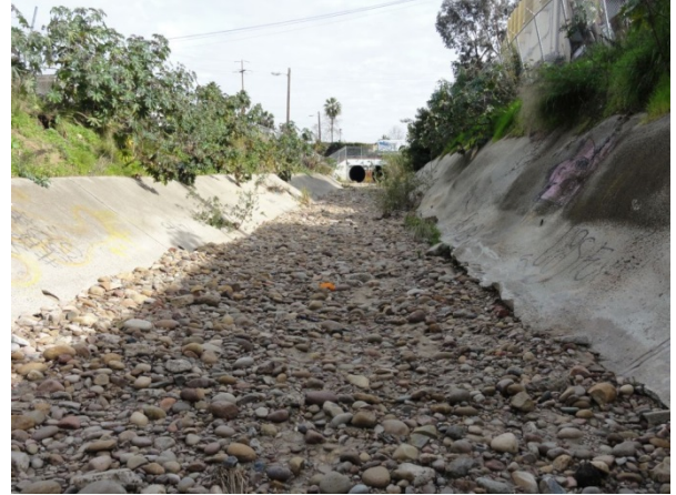
Reach 5 viewing north-east (upstream). Concrete lined side slope on northeast side of channel, and shotcrete side slope on southwest side of channel. Note cobbles, channel is generally clean.
