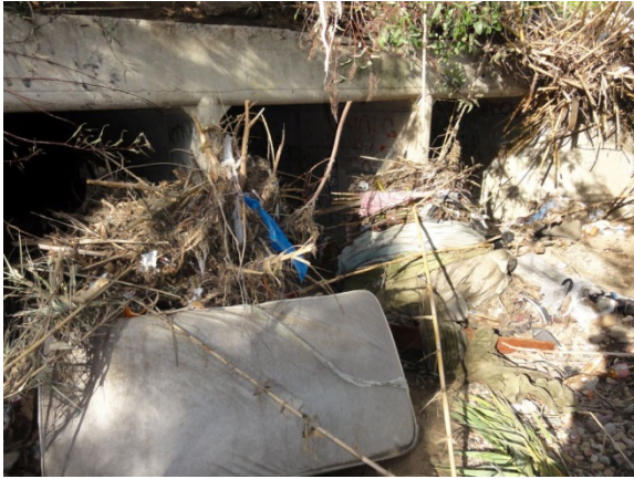
Downstream portion of Reach 1 viewing north-west (downstream) at the triple 6-ft. by 6-ft. box culvert under Spillman Drive. Photo shows 50% clogging of box culvert.
