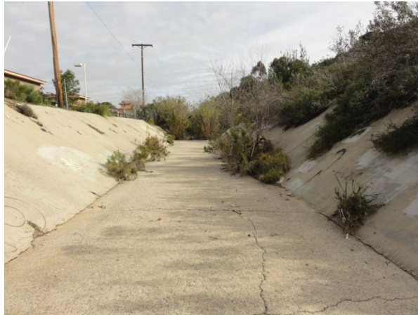
Concrete lined Reach 3, viewing north-east (upstream) at the channel.
