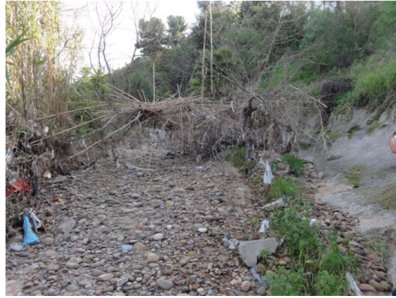
Upstream portion of Reach 1 viewing north-east (upstream) at channel bend. Note dense vegetation and cobble bottom.
