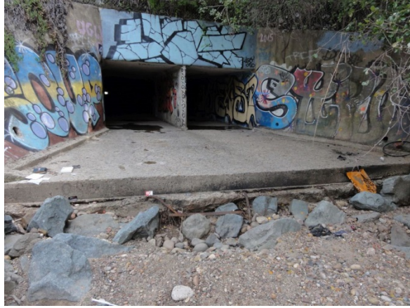
Upstream end of Reach 2, looking northeast (upstream) at 7 ft. by 6 ft. double box culvert. Note rip rap displacement and erosion at concrete apron.
